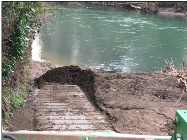
Boat Ramp Silt Removal: With storms subsiding, water levels have dropped, allowing the crew to start the process of removing silt and debris from the launch ramps.
