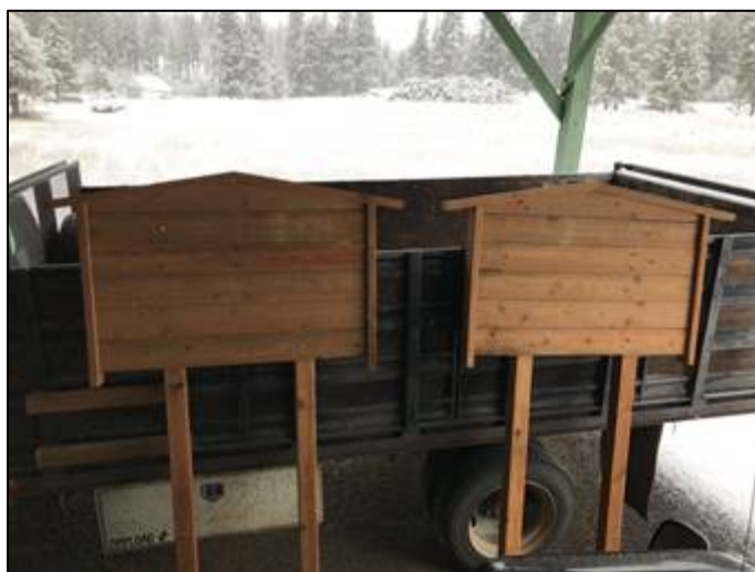
Reader board construction
