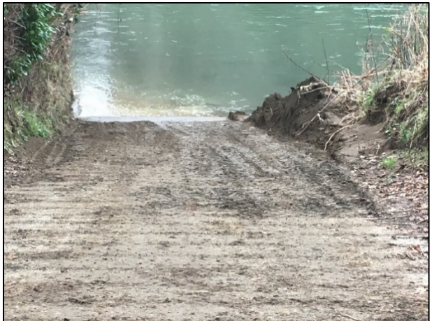
Boat Ramp Silt Removal: With storms subsiding, water levels have dropped, allowing the crew to start the process of removing silt and debris from the launch ramps.
