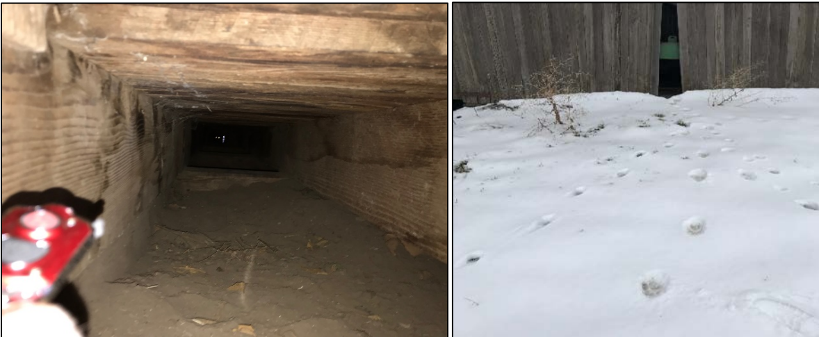
Area under the barn and tracks leading to the crawlspace
