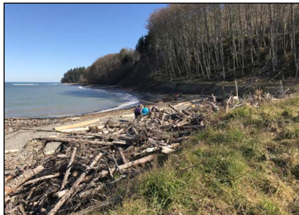
West Twin River target property; this view is east of the “mole”
