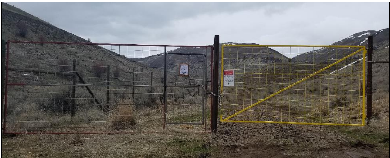
Black Canyon gates after installation on new walk-through gate
