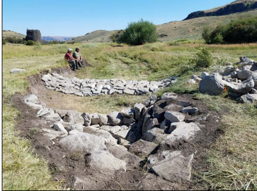
Grand Coulee zuni bowl and one rock dam Zeedyk structures – School Creek, Big Bend Wildlife Area
