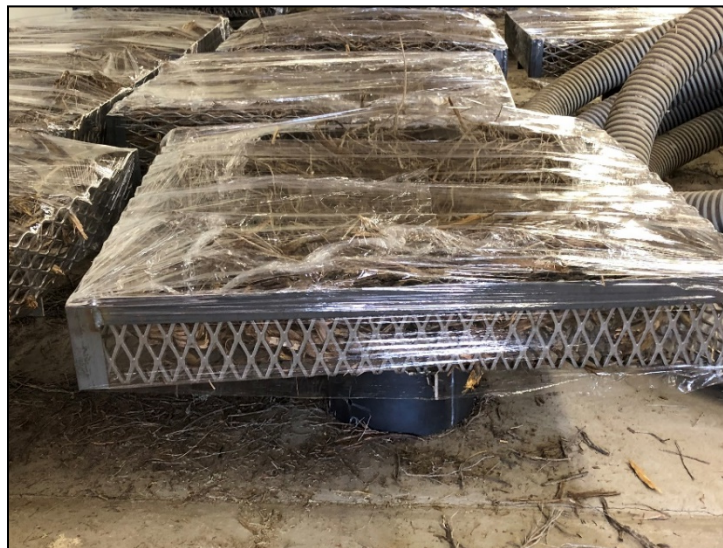
Platforms with sagebrush nest material, wrapped to secure material during installation
