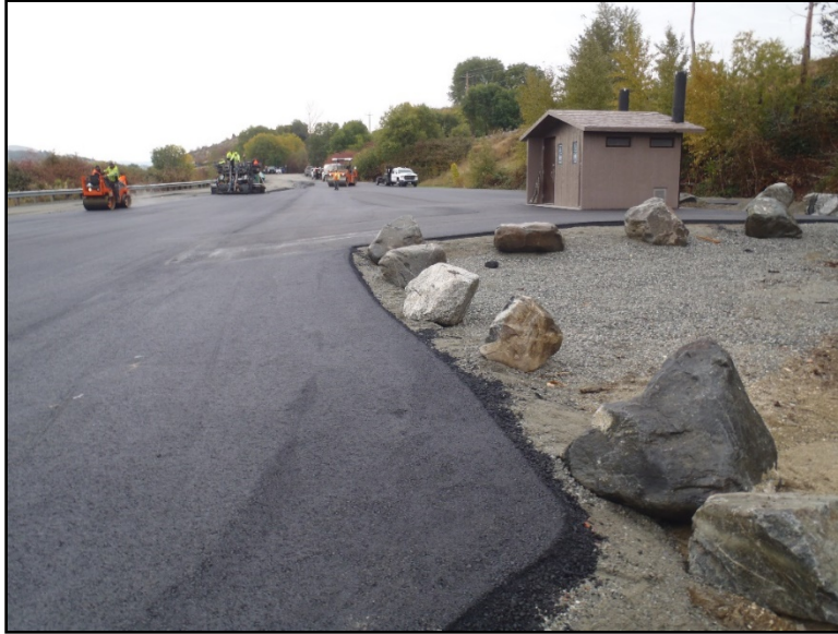
Before and after photos of the access site showing new paved surface throughout and new vault toilet - Photos by Mike DeHart
