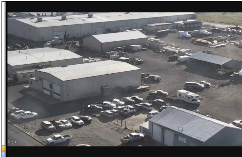
WDFW's Clarkston shop and storage yard as seen from a nearby Port of Clarkston security camera
