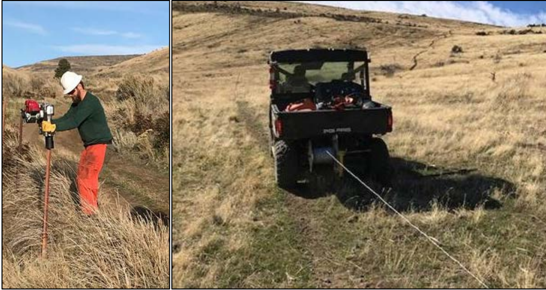
Constructing a riparian cattle exclosure
