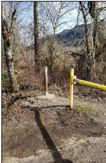
Post to block vehicles driving around the gate
