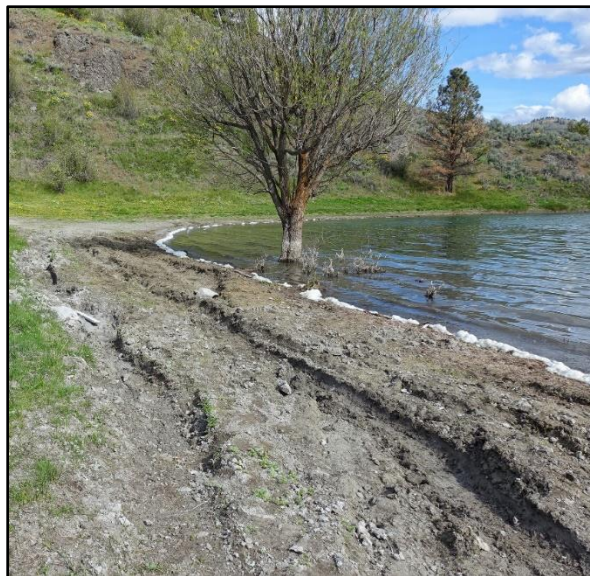
'Mudding' damage during closure on the Blue Lake water access site - Photos by Justin Haug
