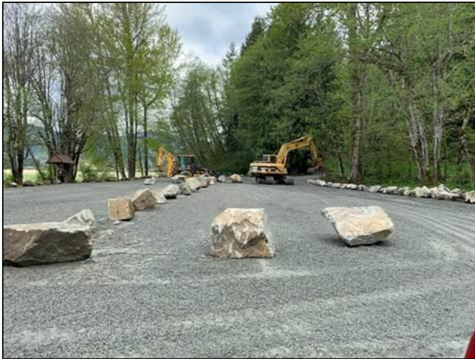
Tacoma Crews repairing and upgrading the Kosmos and Dogpatch parking area
