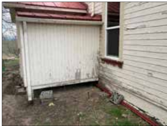
Crawlspace under the house where the cougar was found to be resting
