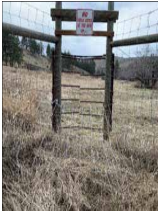
Entry gate panel bent for illegal access during winter closure
