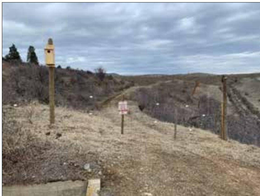
Wire gate with repairs after old posts had rotted away
