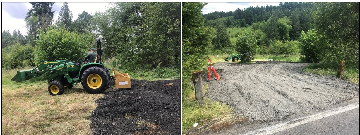
Manager Hauswald spreading gravel and the completed parking area
