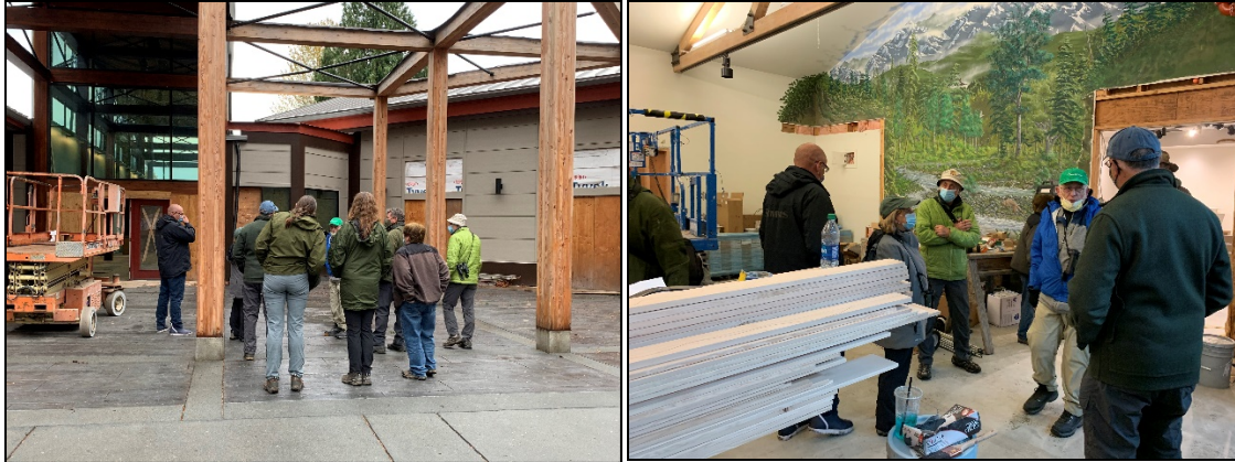
Dungeness River Nature Center (Under Construction)
