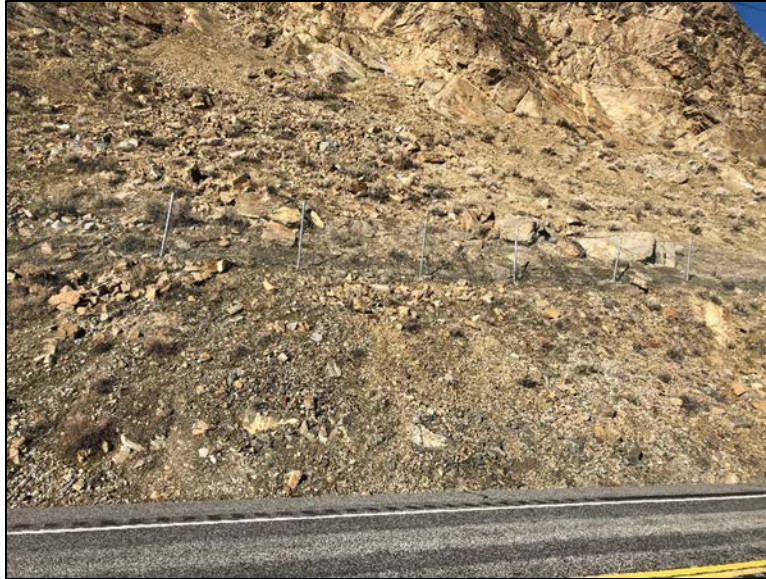
Photos of the completed repairs to the fence
