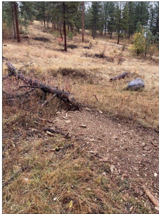
Clearing brush and tree debris with WDFW masticator
