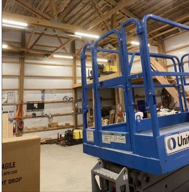
Swakane shop with a newly insulated ceiling, making conditions in the shop much more bearable — Photo by A. Pavelchek
