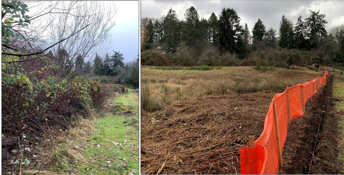
Before and after fence construction progress photos December 2022
