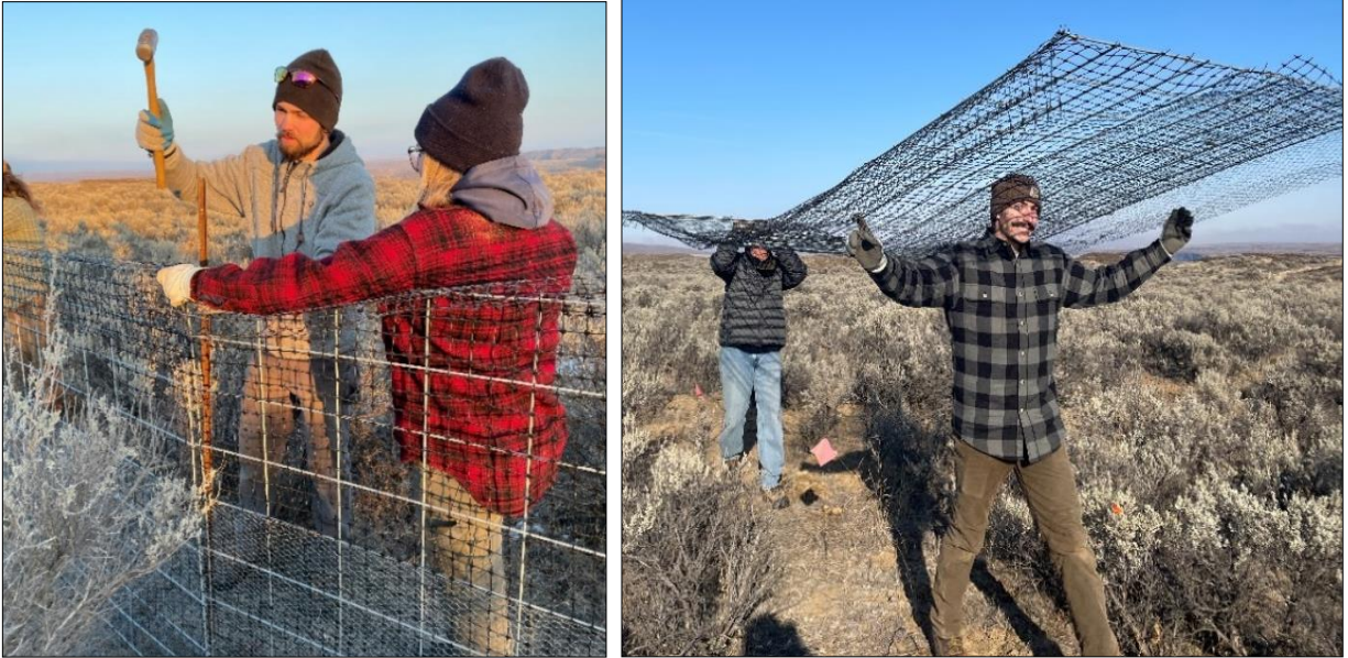
(Left) Washington Conservation Corps (WCC) Crew Member, Jacob, and Crew Leader Emily, drive angle iron into frozen ground (Right) WCC Personnel and Volunteer Carry Fence panels to their destination
