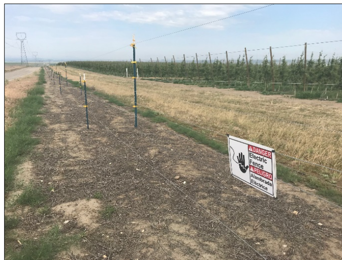
3D electric elk fence in Walla Walla County
