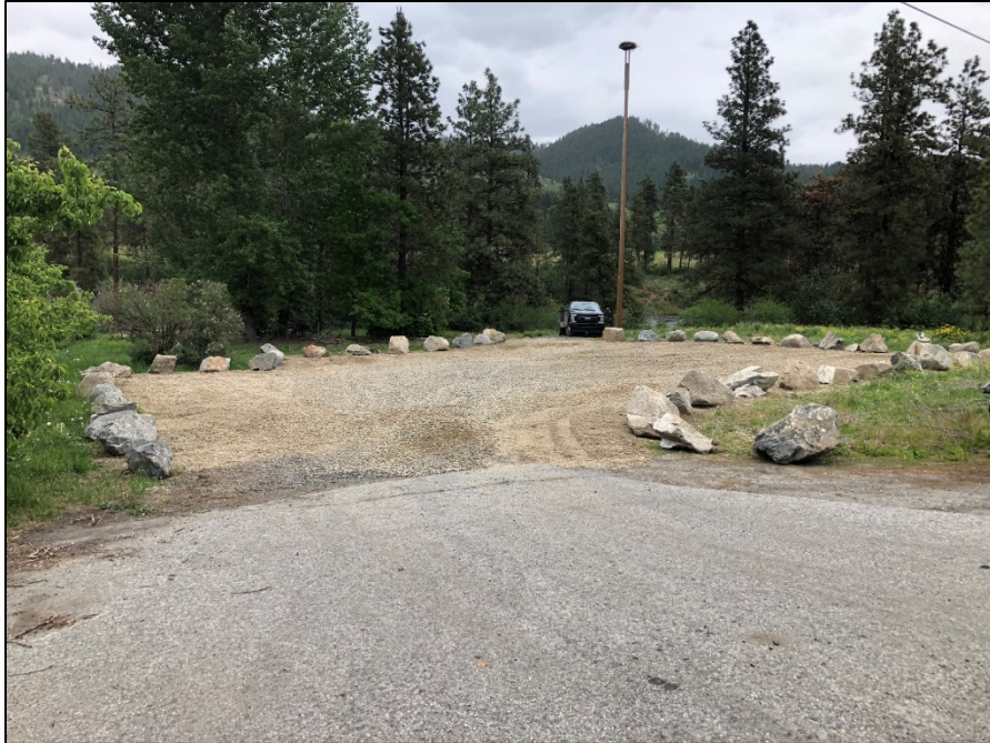
New parking lot at the Leavenworth site - Photo by Josh Harmon
