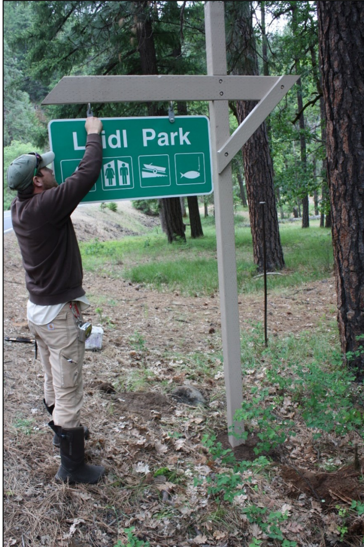
New sign being installed at the entrance to Leidl Park campground
