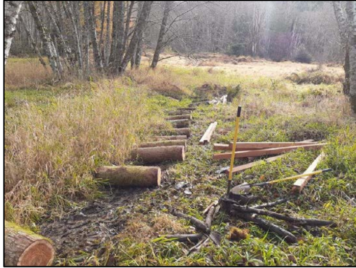
Cedar rounds were used for the footings
