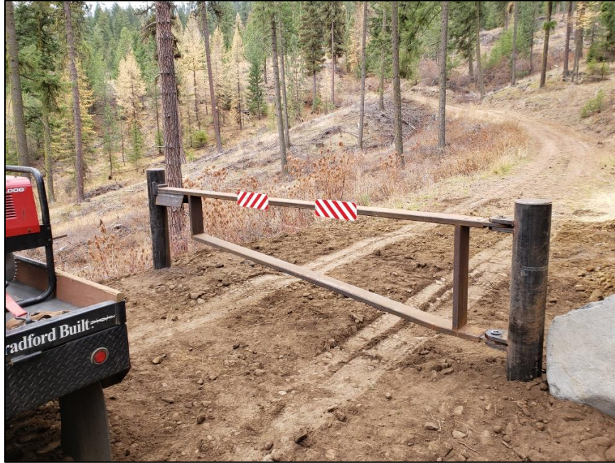
Completed gate installation
