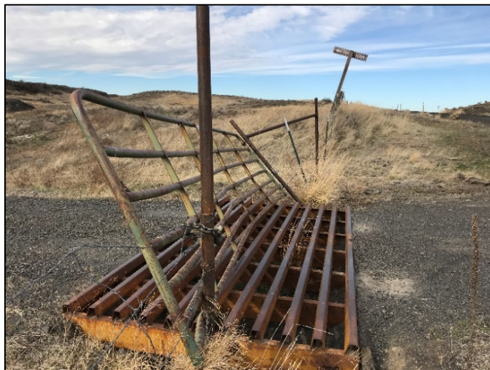
Gate damage, before repairs - Photo by Randall Osborne
