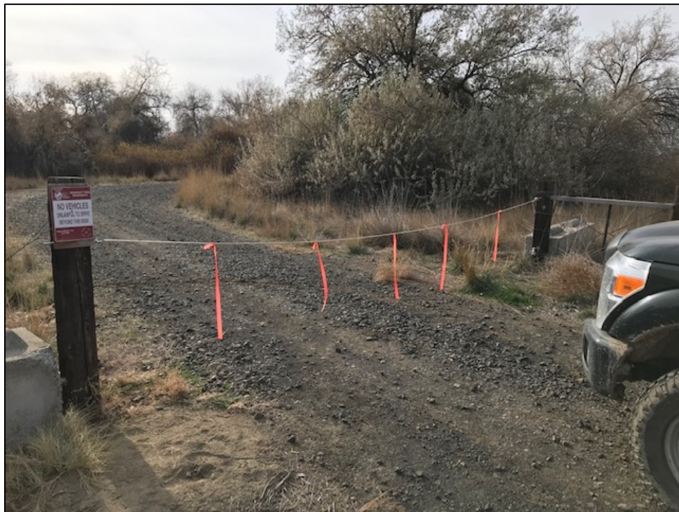
Cable gate installed as temporary measure
