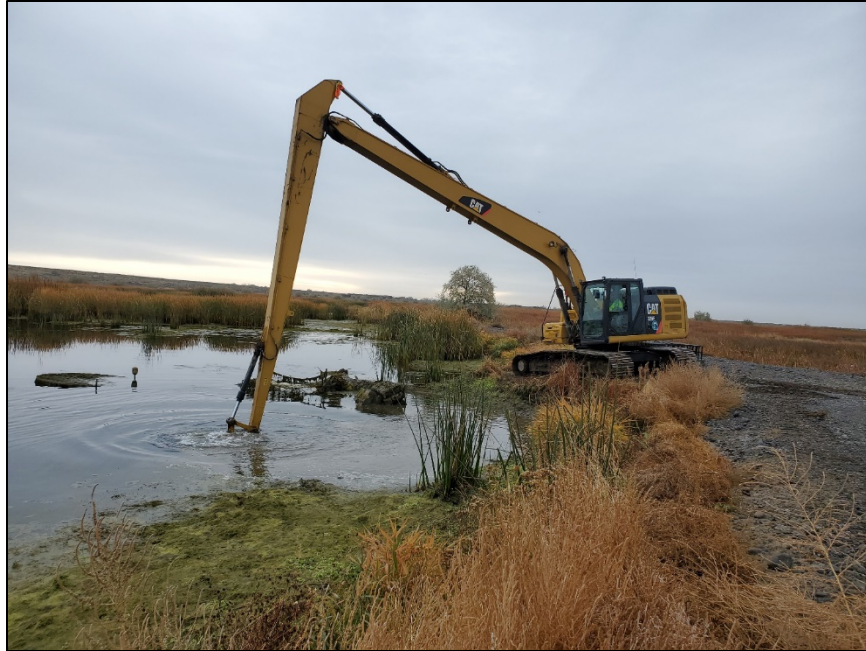
Irrigation operator cleaning out sediment - Photo by C. McPherson
