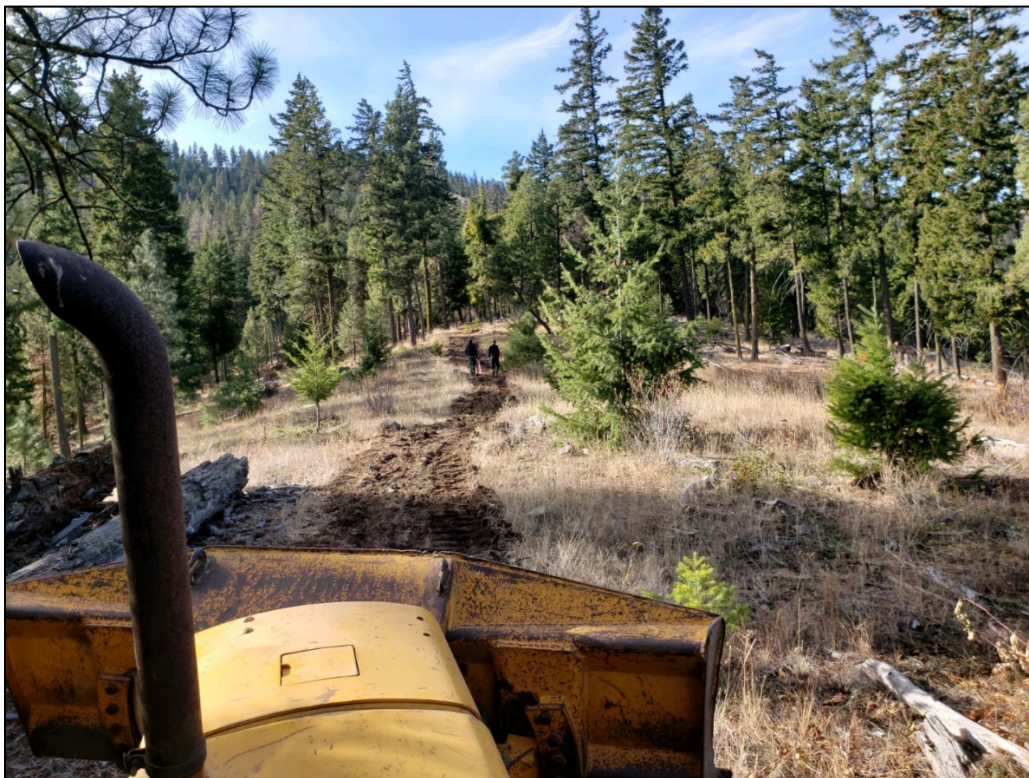
Assistant Manager Berry view of containment line
