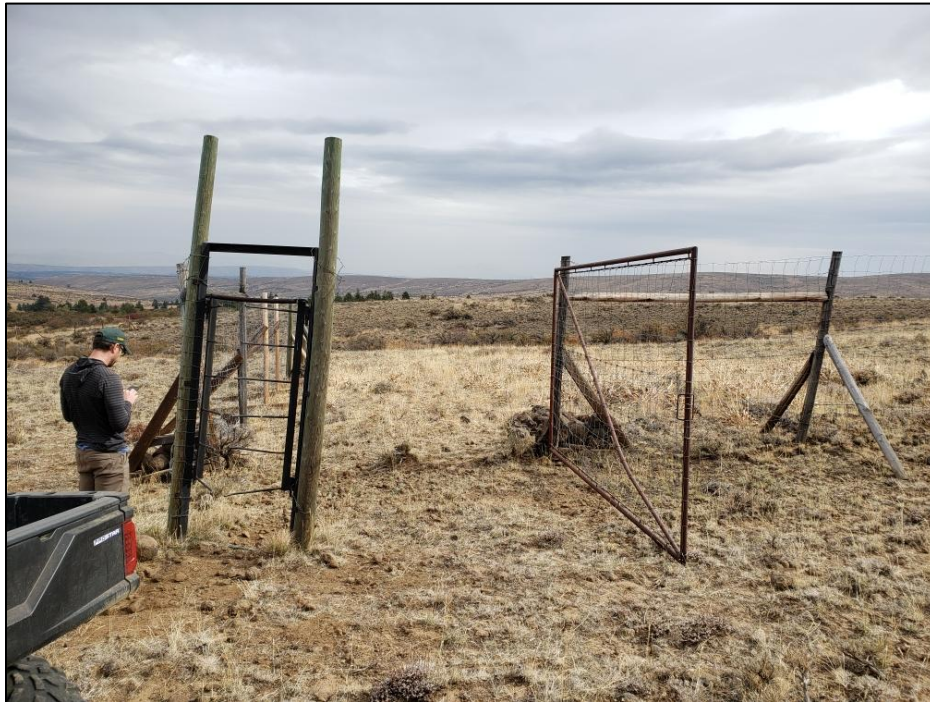
CAMP engineer ground truthing fence location for replacement
