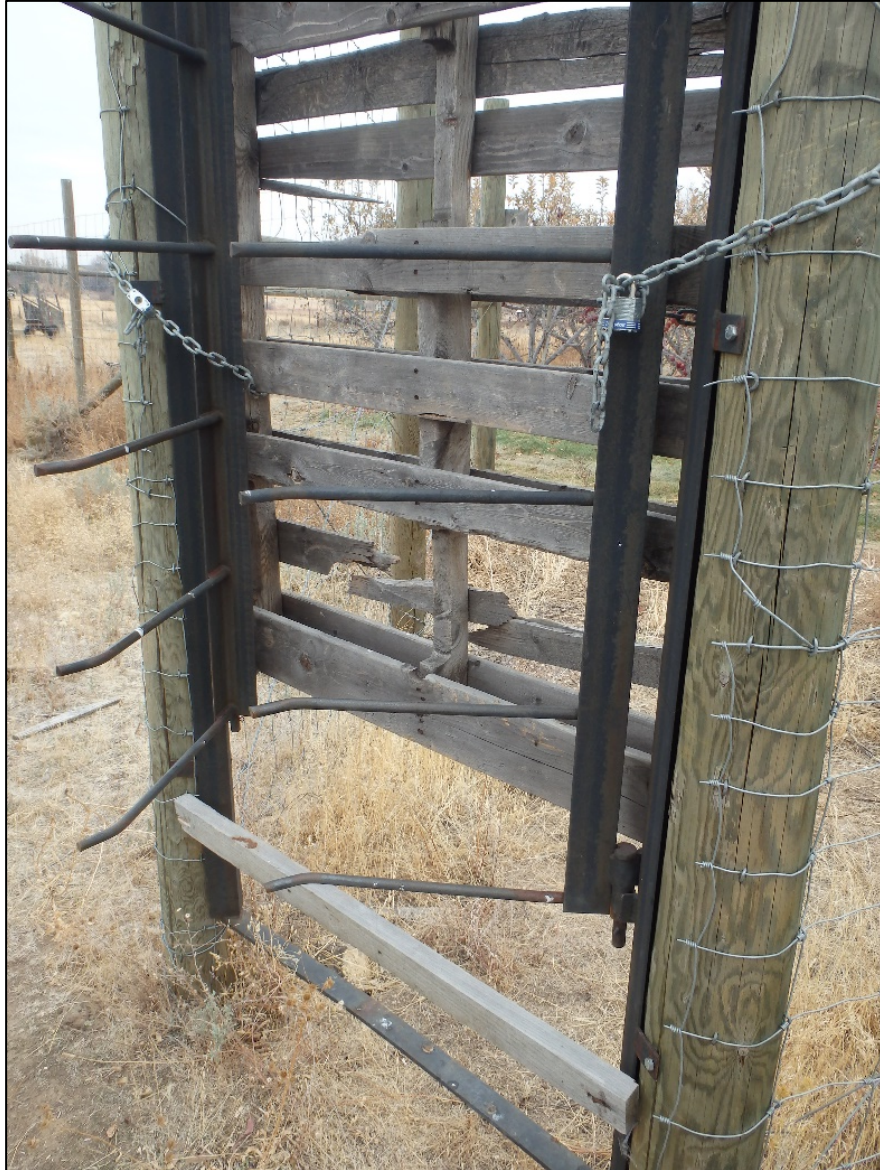
Locked and blocked elk return gate
