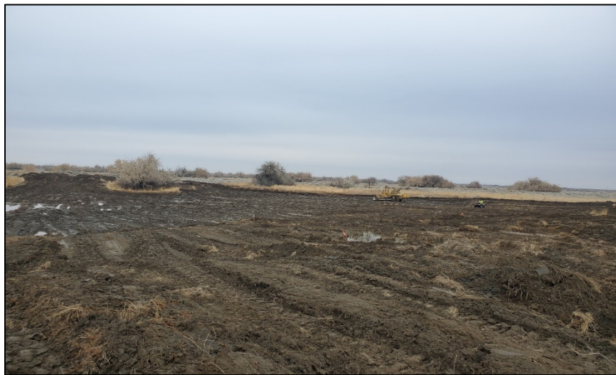
Cat excavating material out of wetland basin - Photo by C. McPherson
