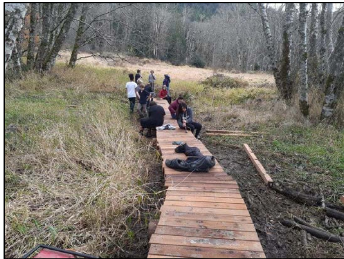
Youth crew decking the new footbridge
