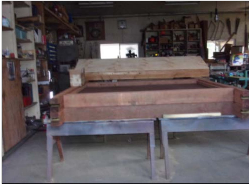
Kiosks under construction at the Olympic shop
