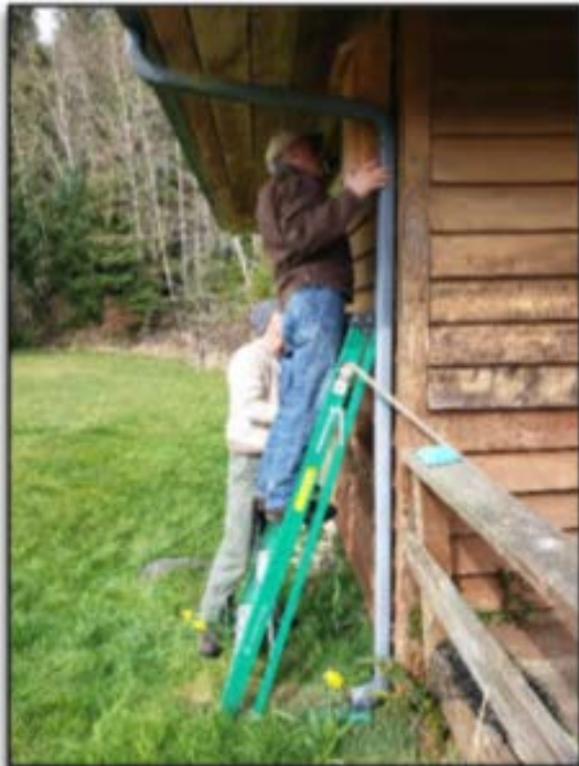
Ryan and Bob installing bat box
