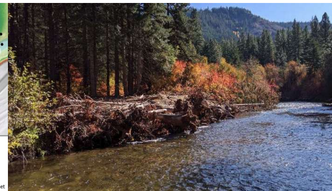
Wood structures buried along the streambank at the project site. (Photo: YN)
