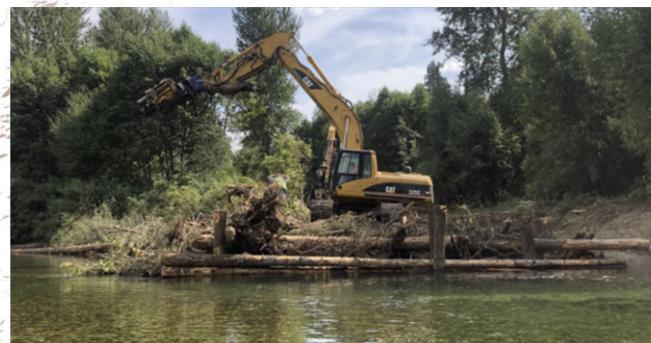
Log structure during construction. (Photo: YN)
