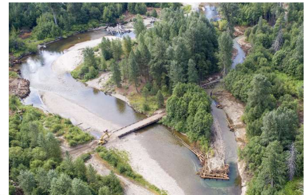
Project in progress, with temporary bridge in place. (Photo: YN)
