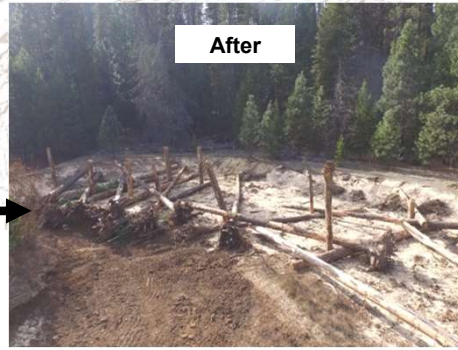
Floodplain reconnected and large wood installed ("after" photo taken before re-watering post-construction).
