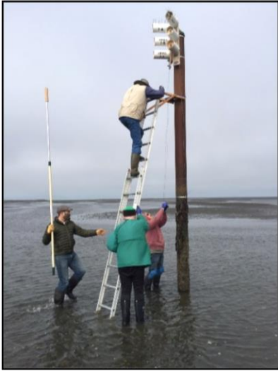
Box installation at Three Crabs - Photo by Laura Davis
