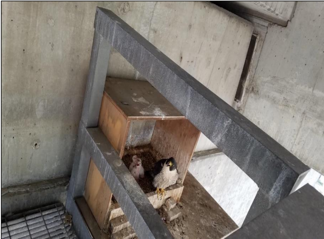
West Seattle Bridge falcon with three eyasses. Workers reported it was not “hello neighbor” at first, which was expected. - Photo by the Seattle Department of Transportation
