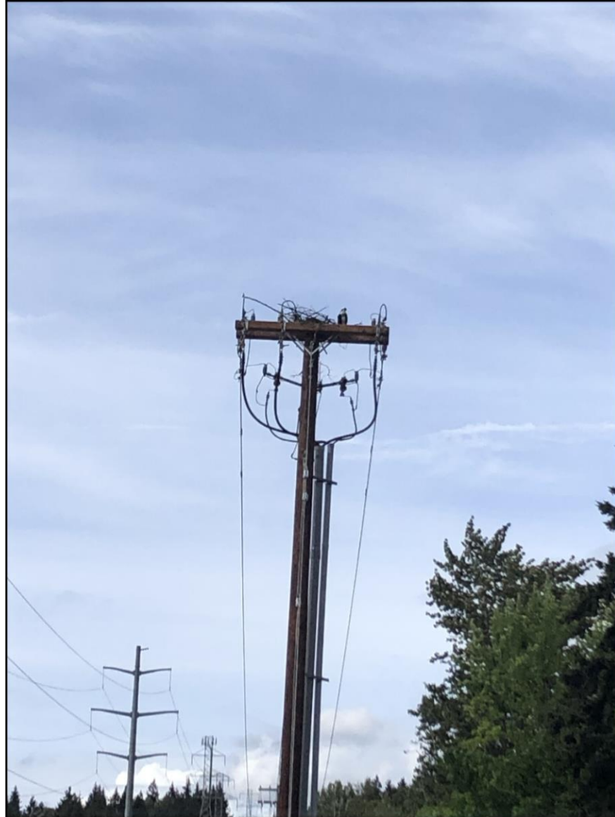
A nest start on a PSE transmission line in Bellevue
