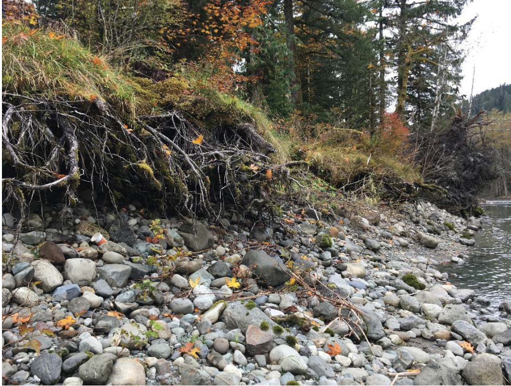
Figure 6. Eroding bank below a campsite within the Gold Basin Campground. The river reroute will start (upstream extent) through this portion of the campground.
