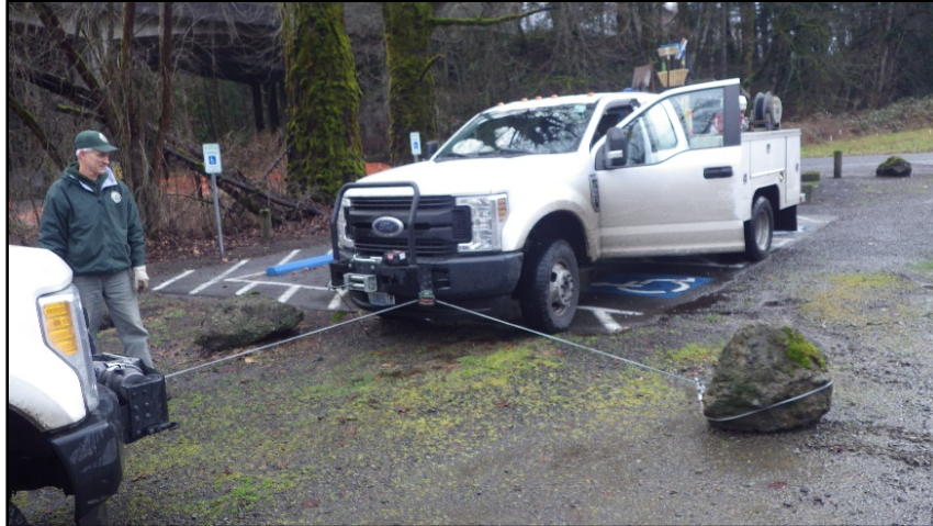
Moving a boulder back into place
