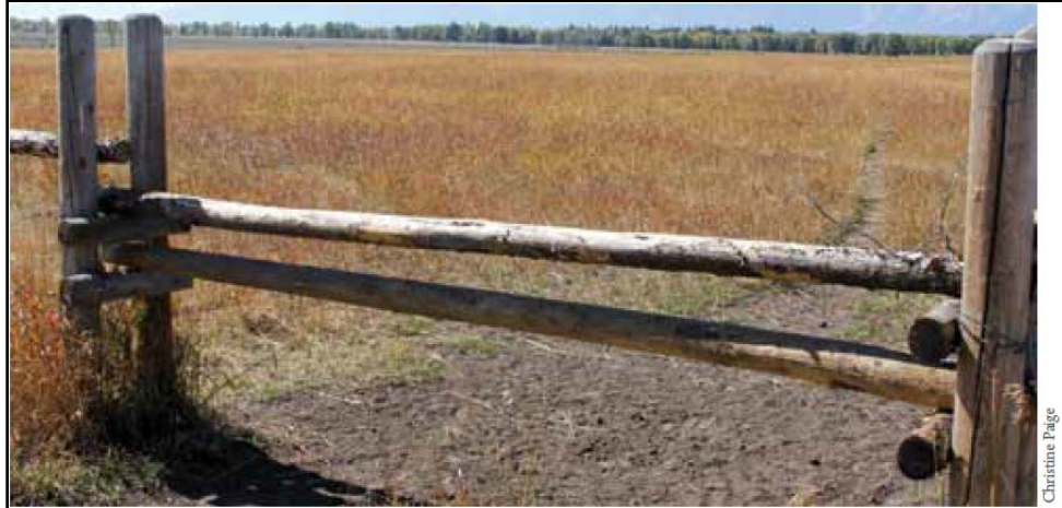
Example of an elk-friendly crossing that Conflict Specialist Jacobsen plans for the landowners to install
