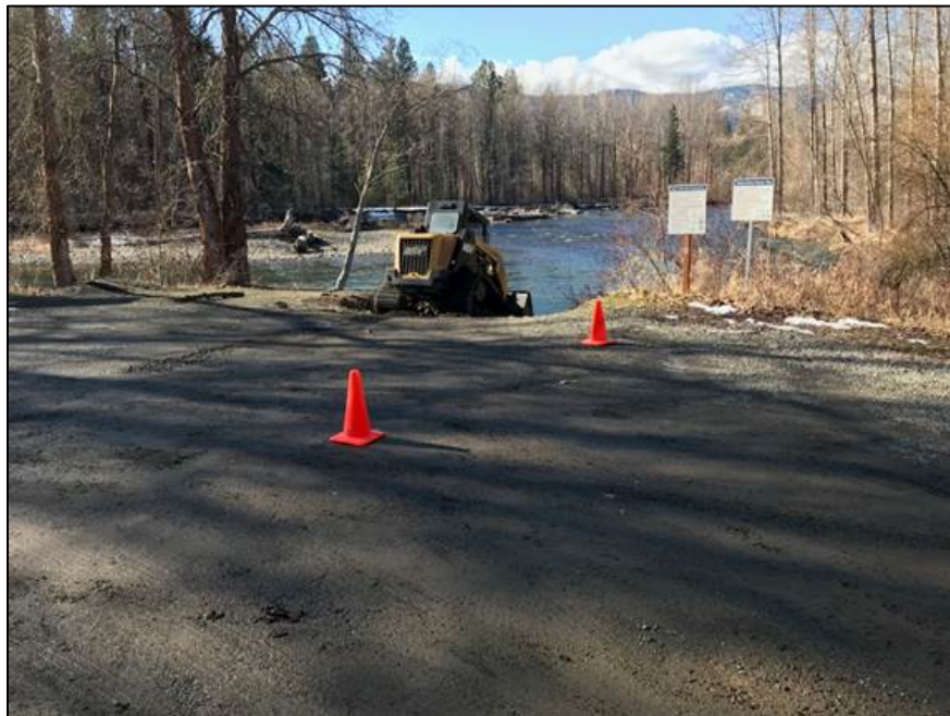
Region 3 Access Area staff members repairing Teanaway Junction primitive boat ramp
