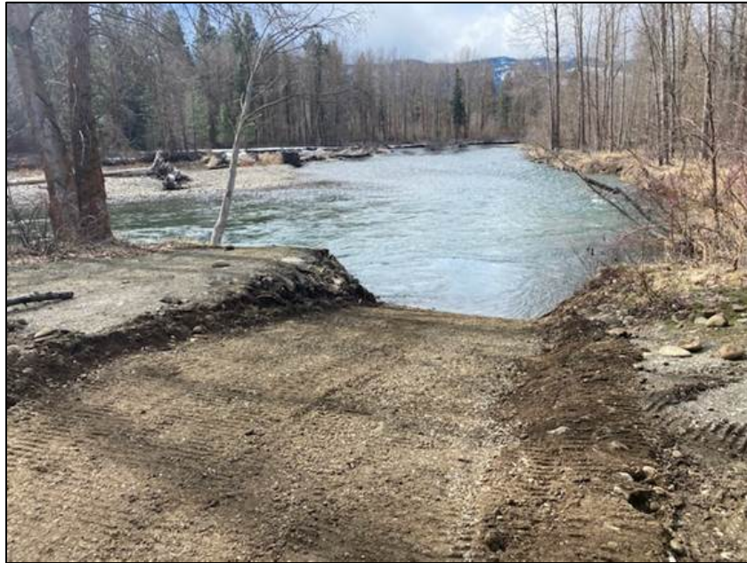
Teanaway Junction primitive boat ramp after being repaired
