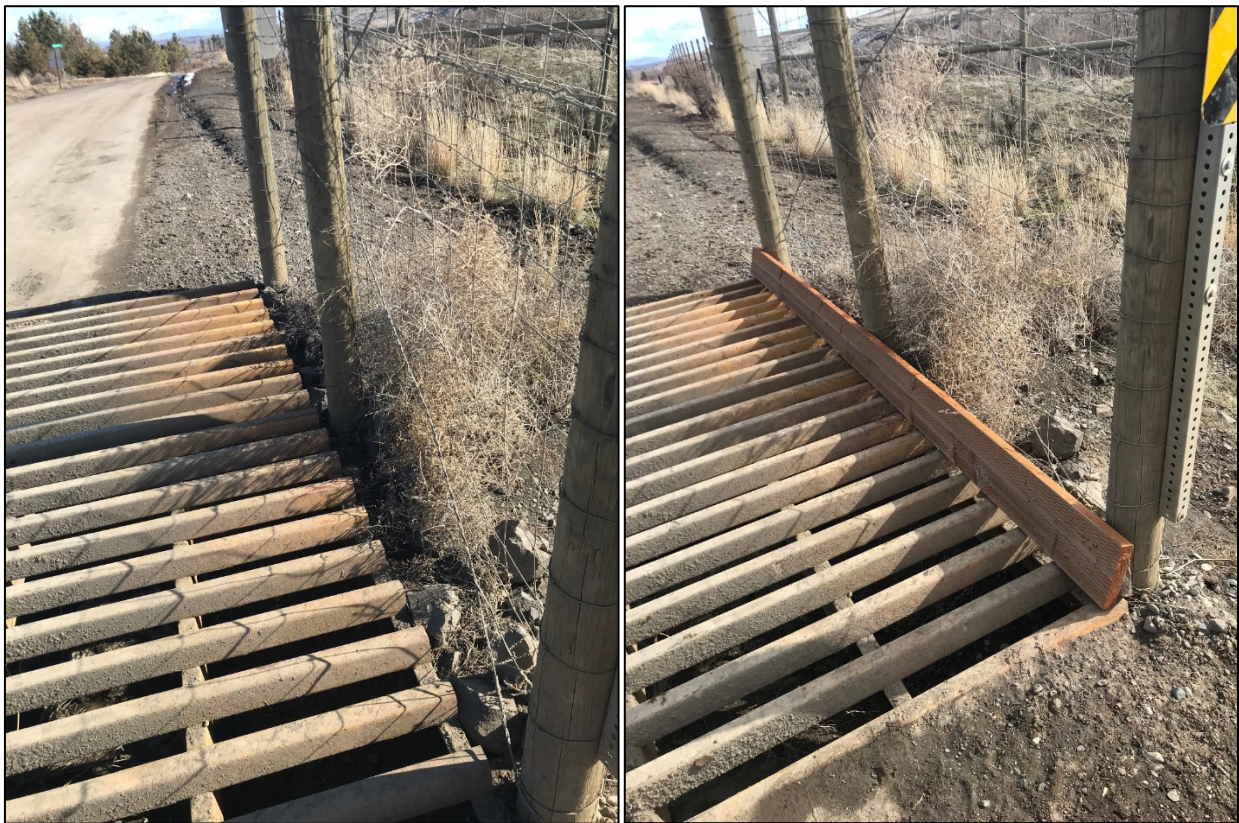
Side plank used to keep elk from using the side of the cattle guard to cross; Elk eventually switched to walking down the center of the grate
