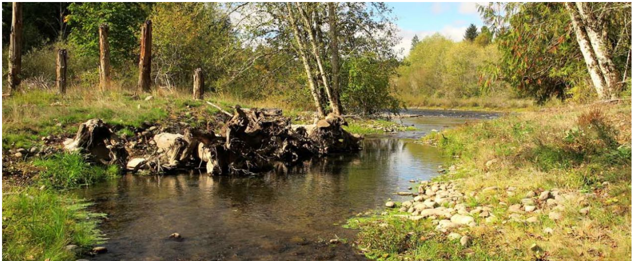
Figure 11: Example of a wood structure in a side channel. Large wood structures in side channels influence geomorphology to help maintain initial side channel geometry along with providing habitat complexity over a range of flows. | Clackamas River, OR
