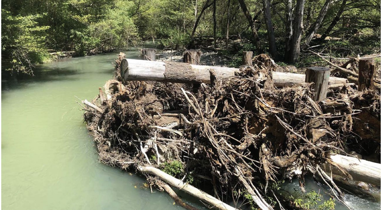
Figure 10: Example of an apex large wood structure at the head of a forested island. The Apex large wood structure influences the geomorphology to help promote and maintain flow down side channels along with providing deep pool habitat at its front and sides. | Dry Creek, CA
