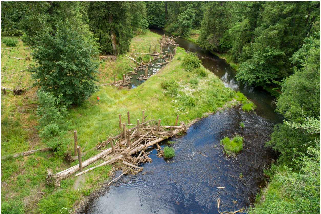
Figure 21: Example of off-channel habitat with large wood placements | Clear Creek, OR
