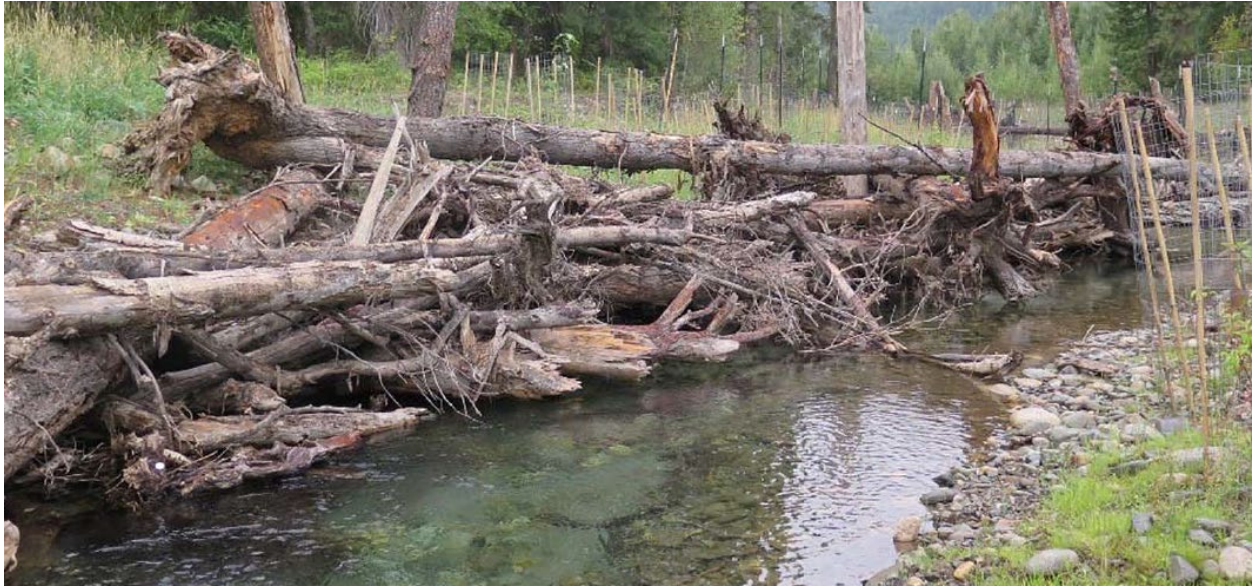
Figure 12: Example of a bank wood structure in a side channel. The large wood structures along channel banks and in side channels influence geomorphology to help maintain initial side channel form along with providing habitat complexity over a range of flows. | Methow River, WA
