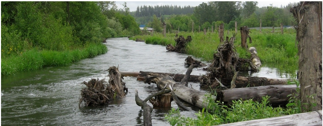
Figure 13. Example of a large wood structure installed to maintain scour pools and encourage side channel formation and floodplain reconnection | Whatcom Creek, Whatcom County, WA
