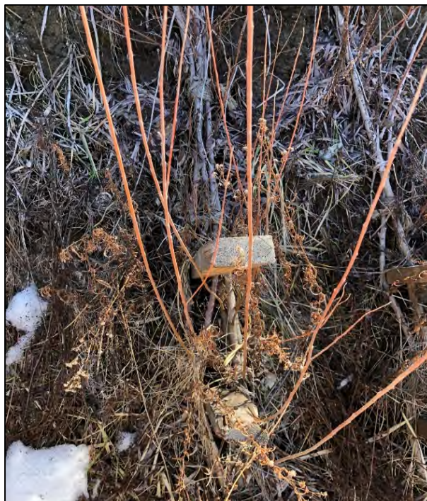
A willow bundle laid in the soil of a cut bank along Tonasket Creek on the Charles and Mary Eder Unit in spring of 2021 to provide bank stabilization. Despite, drought conditions, the bundle propagated – Photo by Dupont
