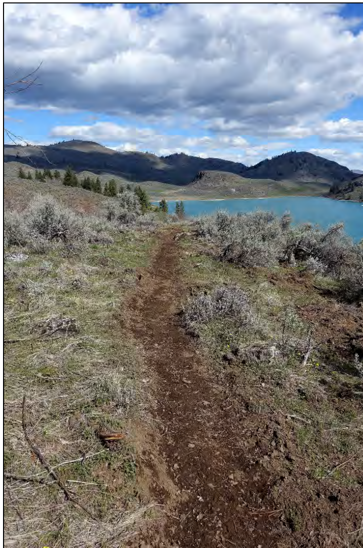
Newly constructed Blue Lake (Oroville) trail – Photo by Haug
