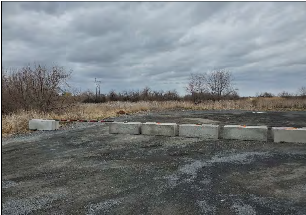
New barrier and gate at road 7 parking area – Photo by C. McPherson
