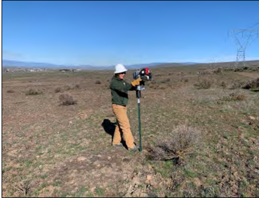
Nass installing t-post around seeded area at Green Gate Subunit
