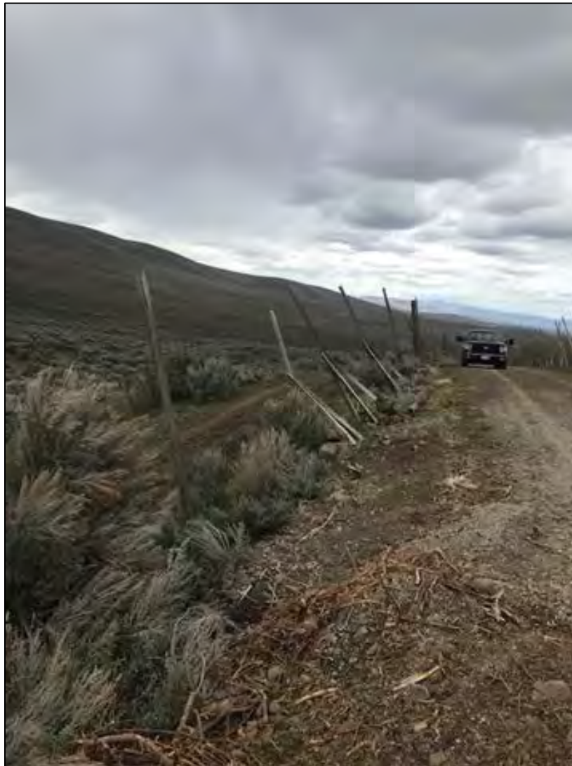
Section of failing rock jacks on elk fence north of Tampico
