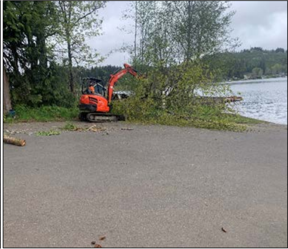
Removal of danger trees
