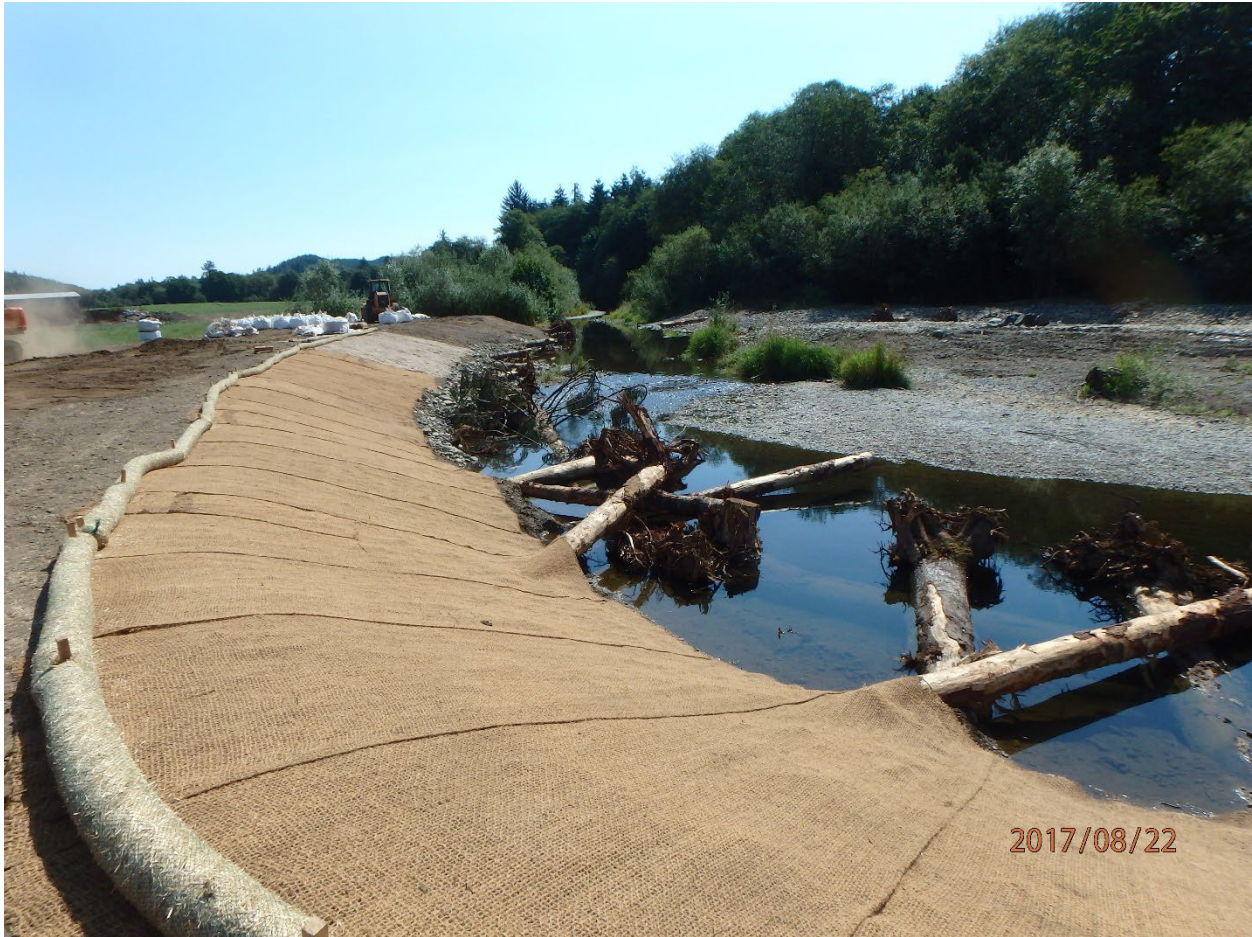
Figure 1: bank protection installed at area 3 as part of phase 1, looking upstream.
