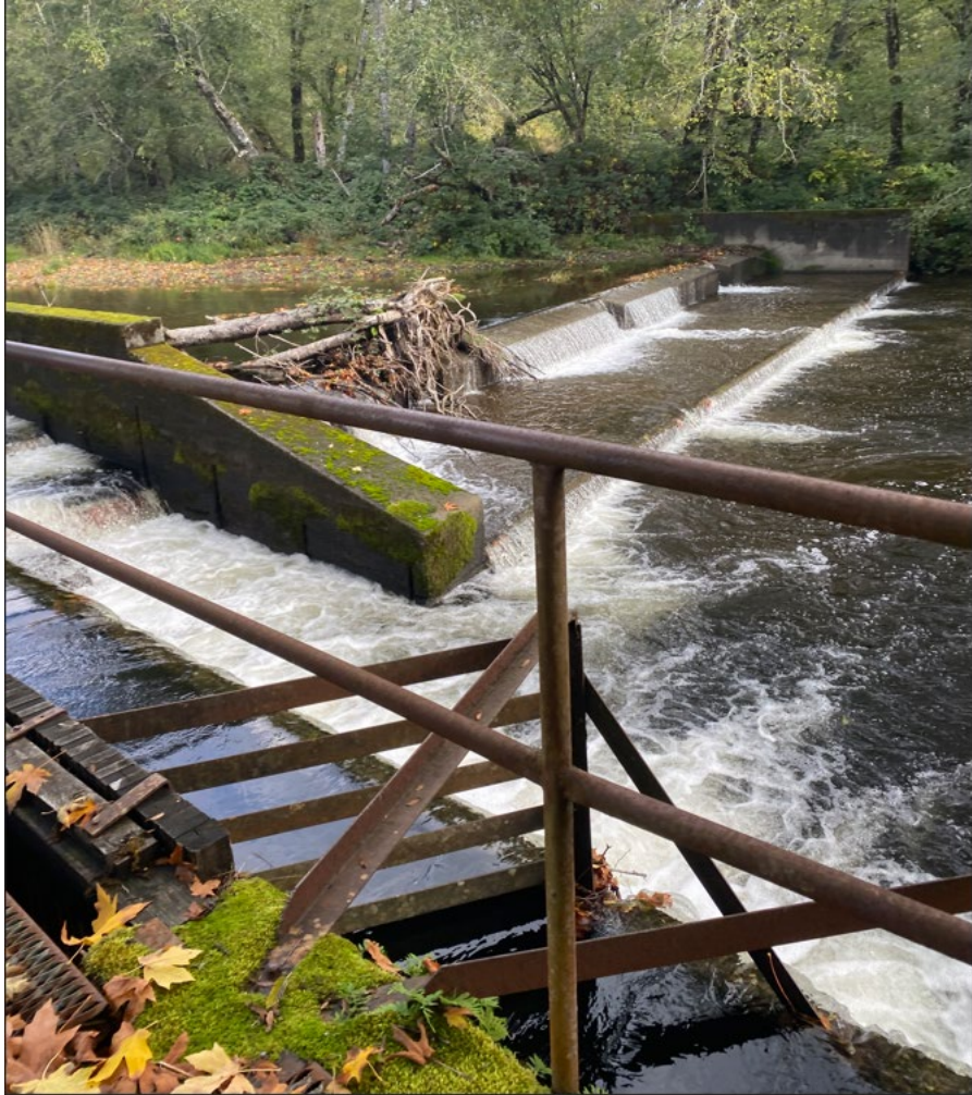
Figure 7: Existing upper intake (area 4, phase 5), showing fish ladder (near) and non-passable weir (far) at moderate flows.
