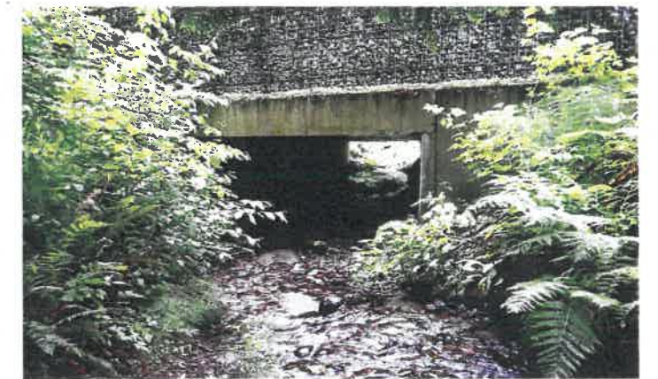
Fish Passage Restoration in a rural environment - SR 531 Cougar Creek
