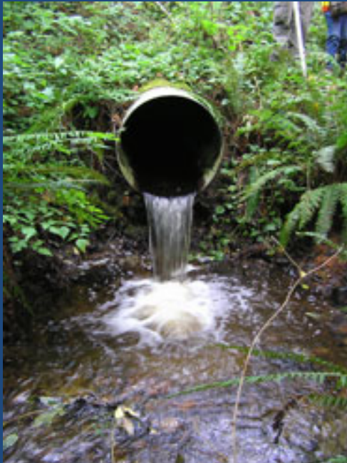
Before 0.7 meter (2.5 ft)
