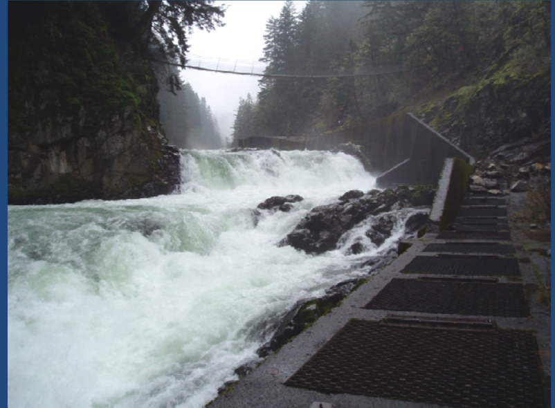
Granite Falls Fishway
