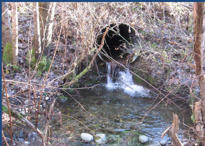
Before: 3 ft diameter culvert
