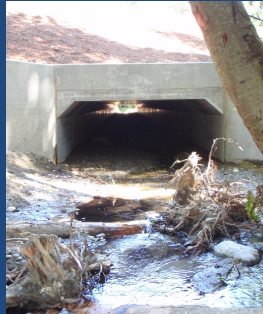
After 3.6 meter (11.8 ft) 3-sided arch
