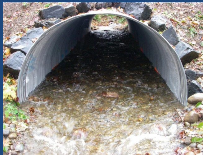
After: 8 ft diameter culvert
