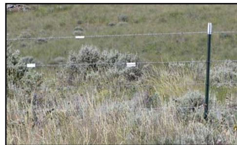
Figure 6. Fence with markers to reduce grouse collisions.
