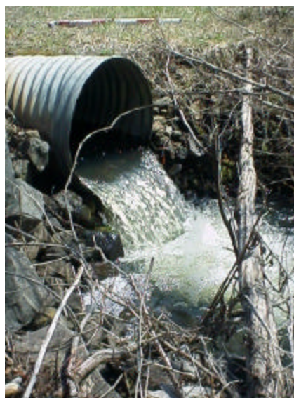
Photo 14. Site T18R16E - 6, on Bear Canyon Creek, is a 0.76 meter diameter culvert, 224 meters upstream of the confluence with NF Manastash Creek. WDNR evaluated this site as a barrier.
