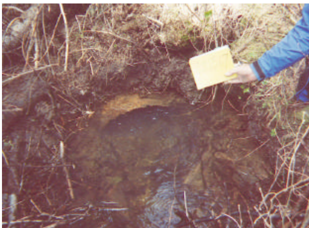
Photo 18. Site 981567, a 0.46 meter diameter culvert. Partial barrier due to slope. Unnamed tributary to NF Manastash Creek.
