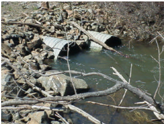
Photo 3. Site 981552 on NF Manastash Creek. Two 0.76 meter diameter culverts are a partial barrier due to velocity and slope.
