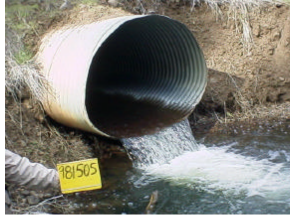
Photo 21. Site 981505, on Robinson Creek, is a 1.75m squash culvert. It is a partial barrier due to a 0.36 m outfall drop and a 4.8% slope. The PI value for this site is 20.71.
