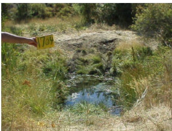
Photo 32. Site 981704 on Quilomene Creek, is a passable ford crossing but unstable banks contribute fine sediments to the stream. This picture was taken after a hunter's truck recently negotiated the crossing.
