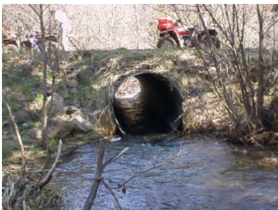
Photo 13. Site T18R16E-12 on Bear Canyon Creek, is a 1.07 meter diameter culvert just 51 meters upstream of the confluence with NF Manastash Creek. WDNR evaluated this site as a barrier. A barrier falls ends anadromous fish access at 1,200 meters upstream.
