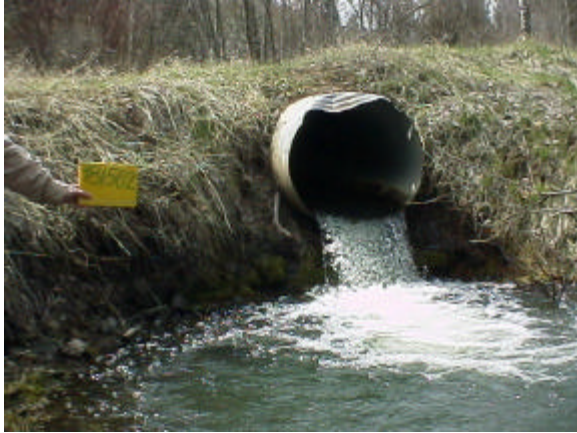
Photo 20. Site 981502 is the first barrier encountered on Robinson Creek in the WLA. This 1.07 m diameter culvert is a total barrier due to a 0.58 m outfall drop, and a 3% slope. This feature has the second highest PI value, 24.20.
