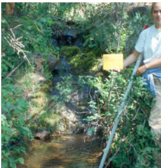
Photo 31. Site 981600 on Morrison Canyon Creek features a dam with an overflow channel 110 m long. This 1.5 m high cascade on the overflow channel is a low flow barrier.
