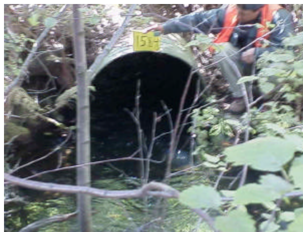
Photo 30. Site 981519, on Shadow Creek, is a 0.91m diameter culvert that is a total barrier due to a 5.5% slope and velocity.
