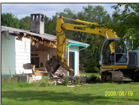
Demolition of old hatchery house for new Spawning Bldg
