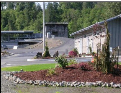
Spawning Building and Fish Separation Facility
