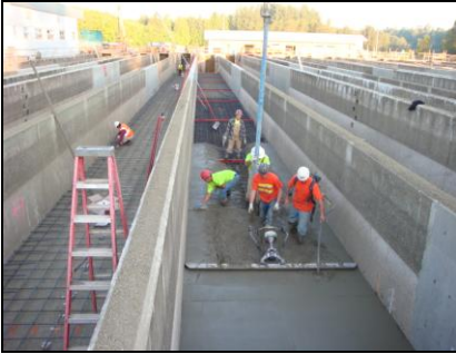
Construction of new juvenile raceways
