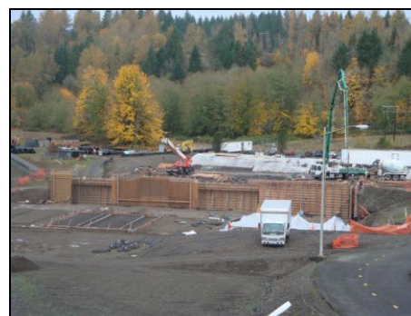
Construction of adult holding ponds
