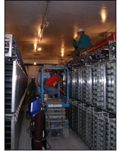
Construction of new Adult Spawning Bldg
