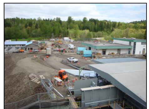
Construction of new Adult Spawning Bldg
