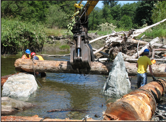
Installing large woody debris jams in Day Creek
