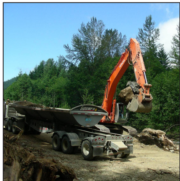
USFS road removal at the Greenwater River
