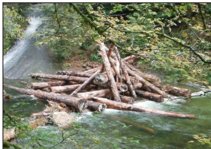
Side View logjam installed at Hardscramble creek
