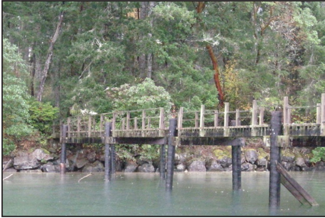
Squaxin Island bulkhead and pier removal - before
