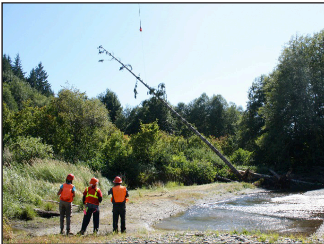
Lower Tahuya River Large Wood Placement August 2011
