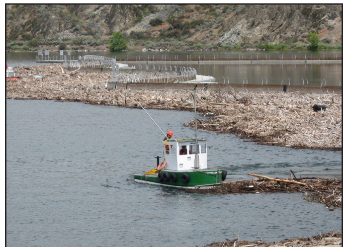
A lot of dam wood. Seen here an annual removal operation at Wells Dam on the mainstem Columbia
