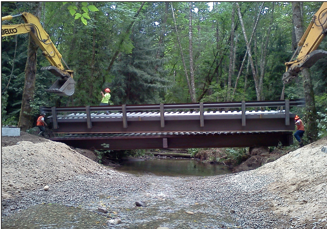
Placing a new bridge at Purdy Creek
