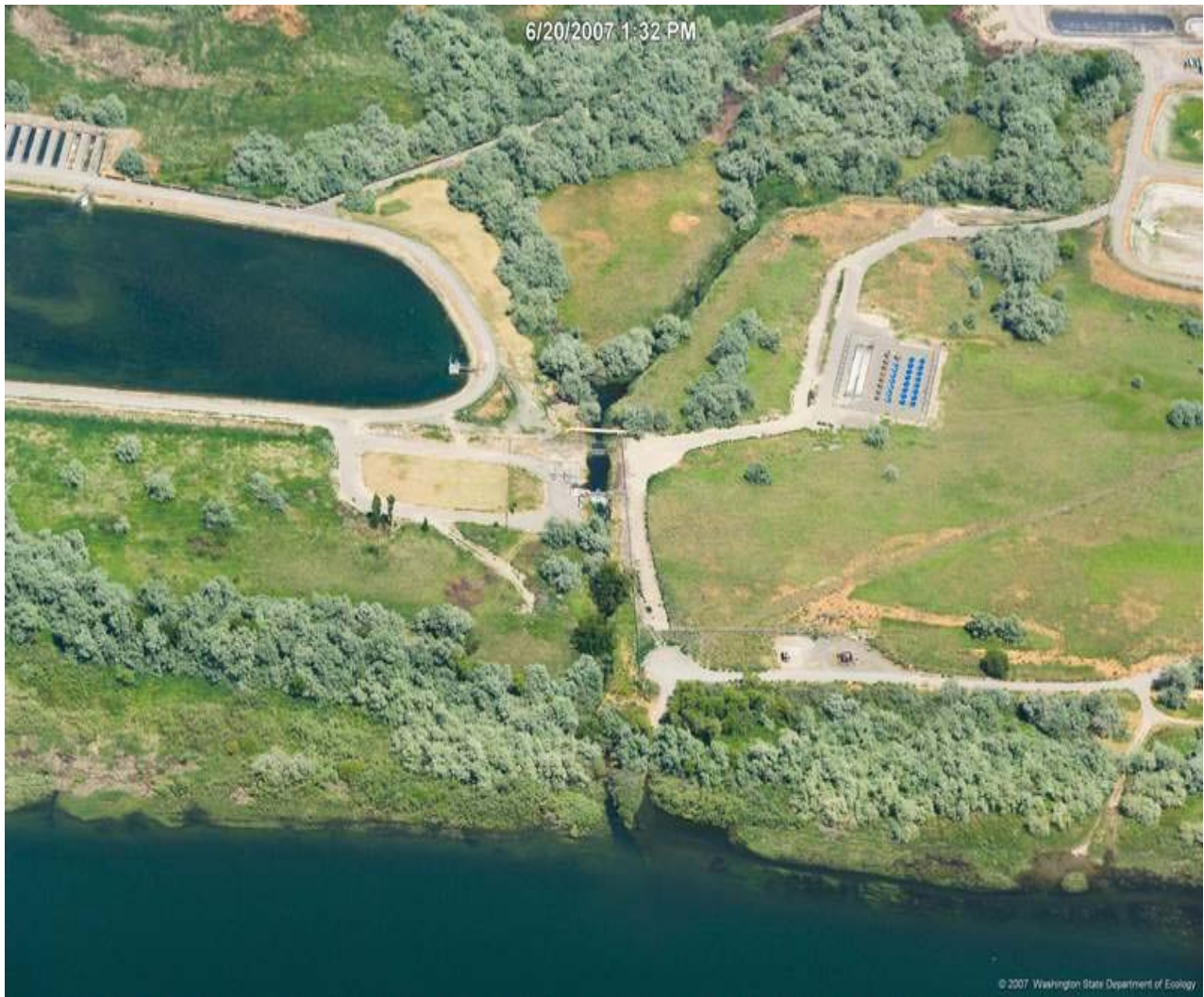
Figure 3. RSRF 9-acre pond, outlet structure, fish trap, 2 concrete raceways and 32 blue round tanks.
