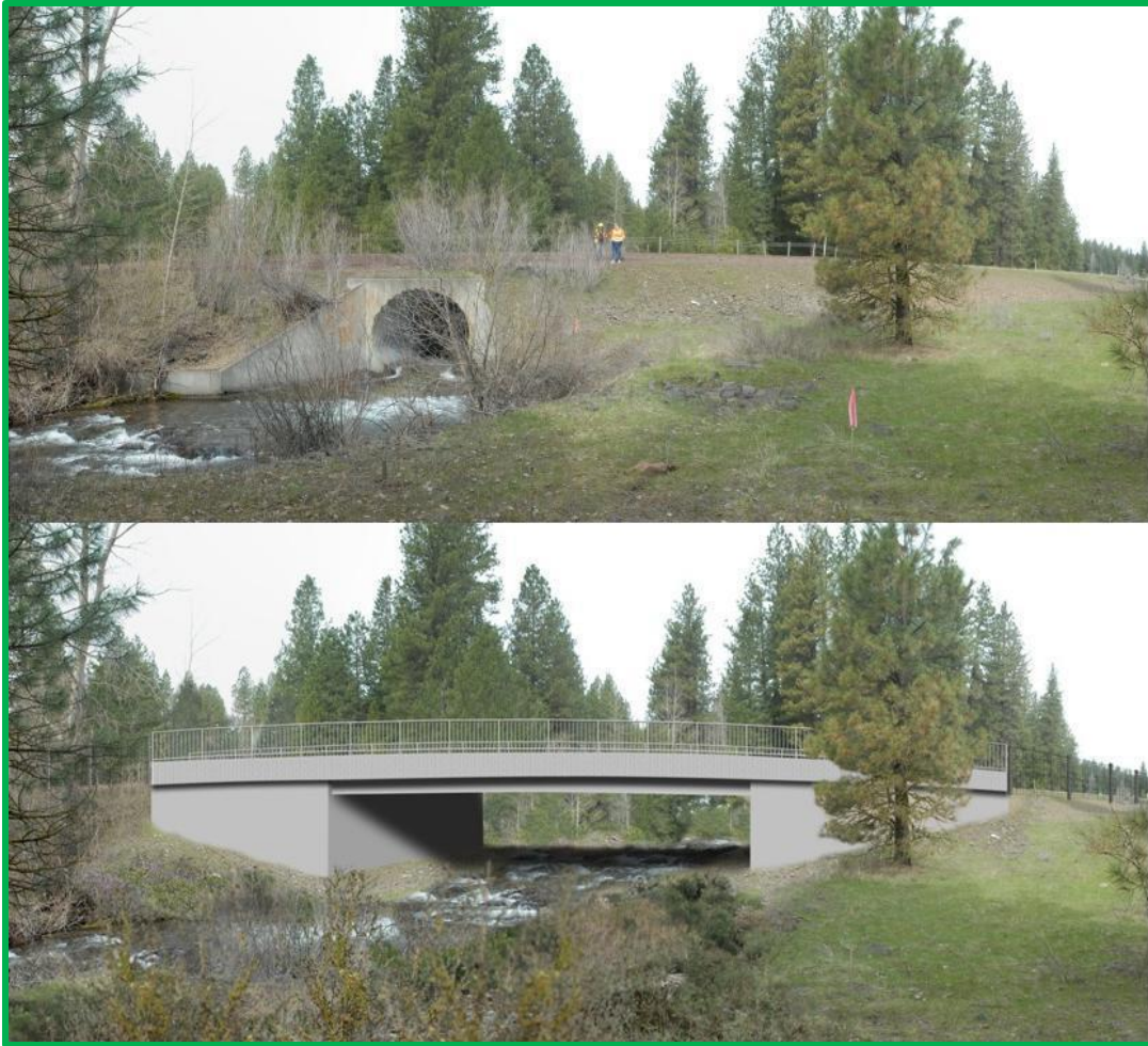
Improved wildlife crossing at Butler Creek on SR 97 north of Goldendale, WA. Photo WSDOT
