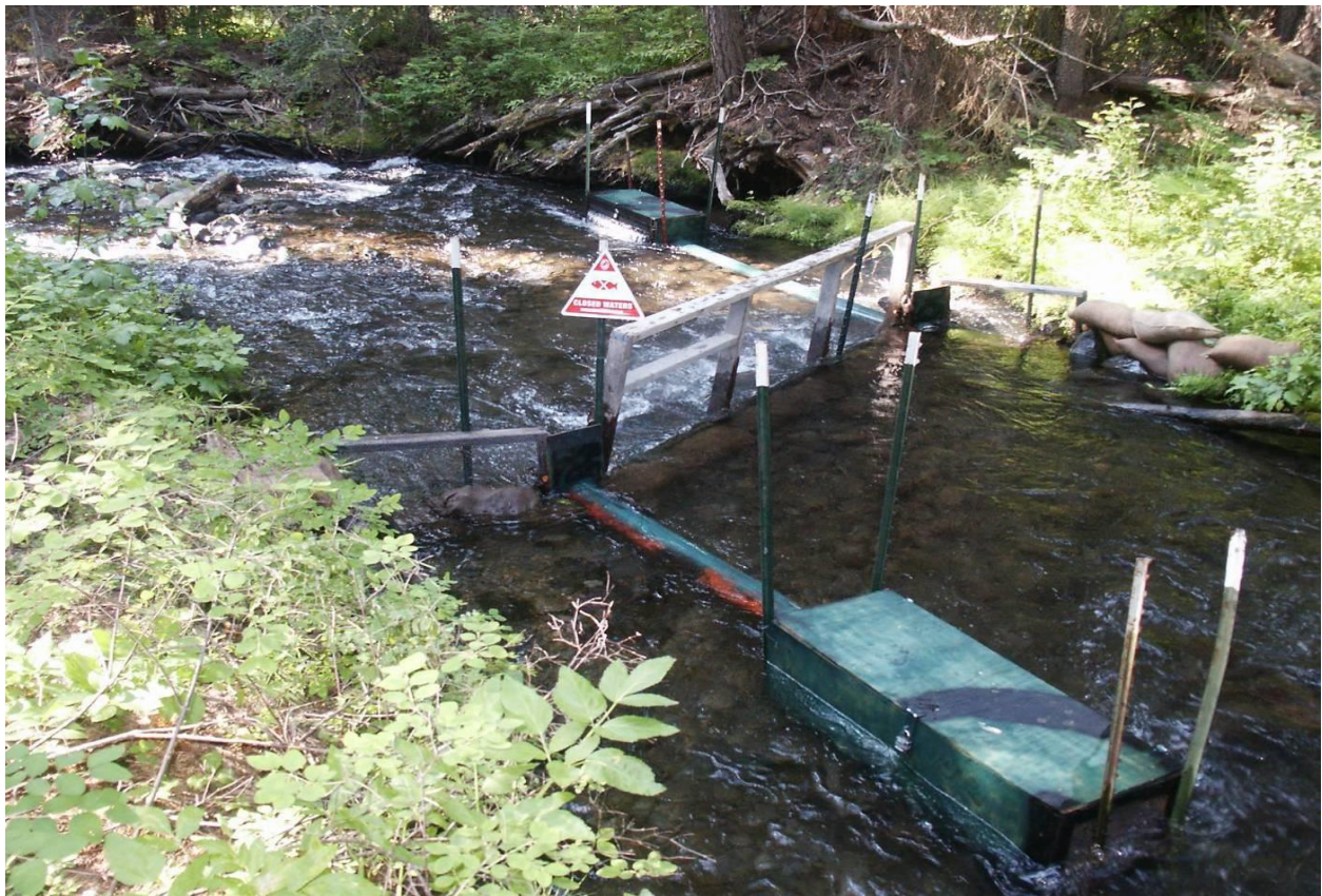
Figure 6. N. F. Ahtanum Creek "N" style weir with upstream & downstream box traps.
