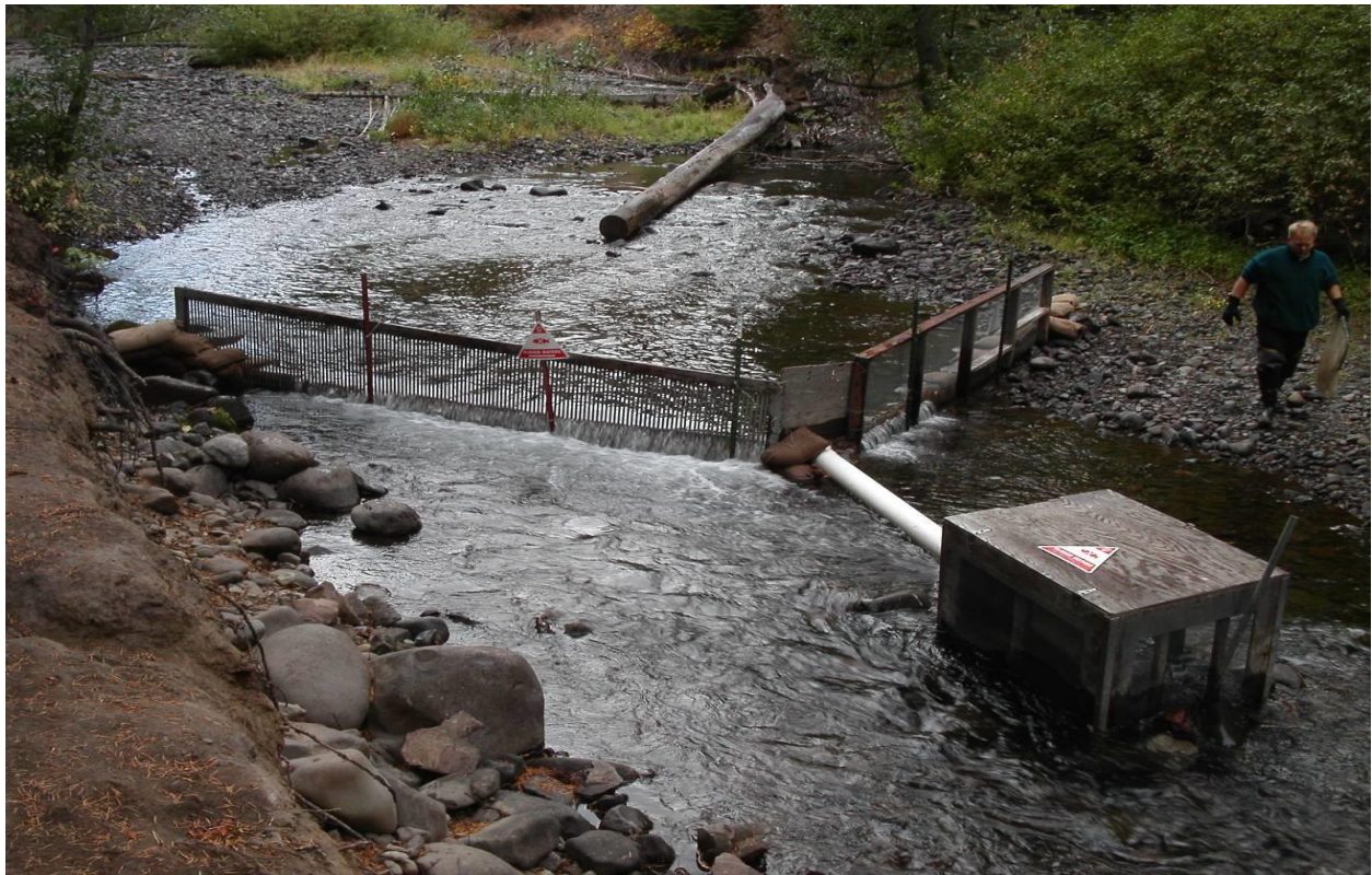
Figure 5. Crow Creek "V" style panel weir with live box trap.
