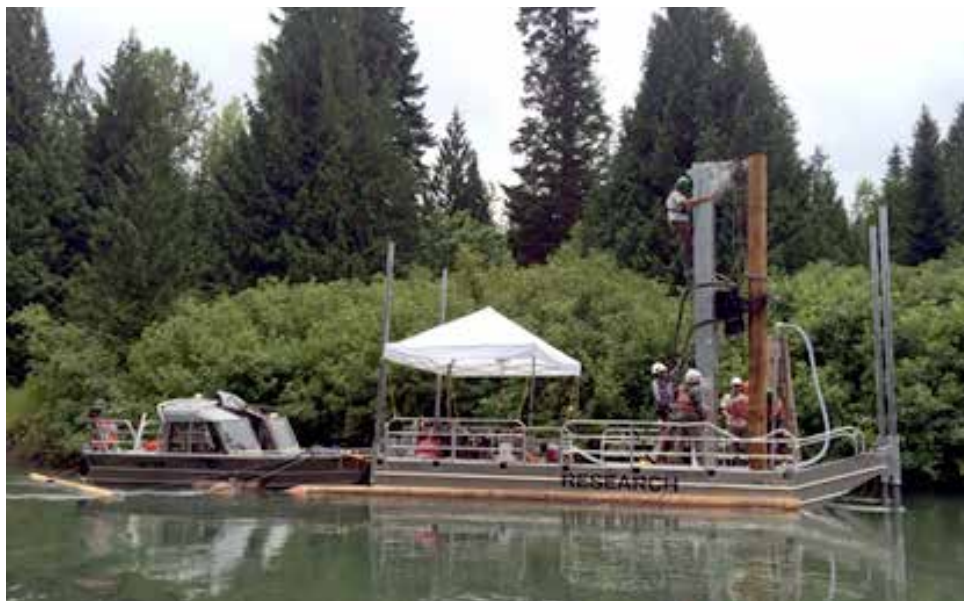
White River Large Wood Atonement Project. Photo by USFWS.
