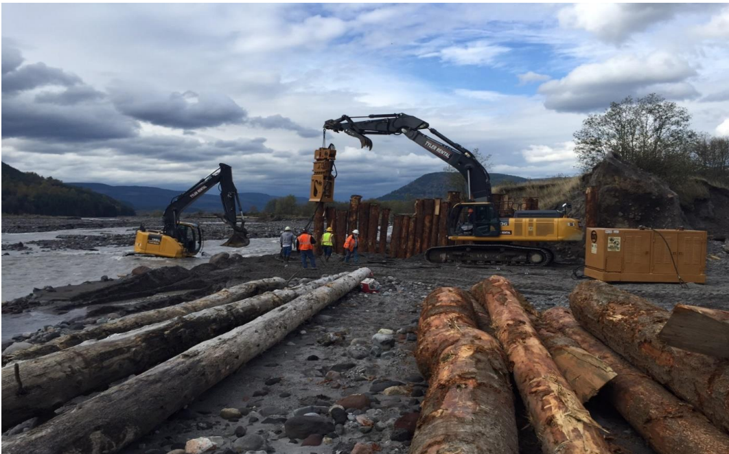
Pile Dike Construction Mudflow Unit. Photo by Daren Hauswald.
