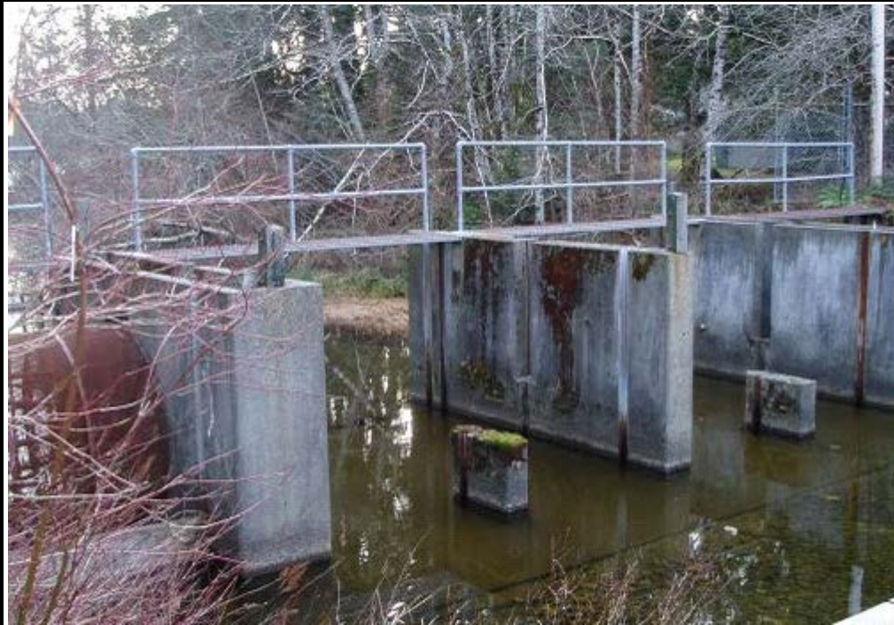
Lake Screen – Screen at the inlet or outlet of a lake or pond, typically intended to prevent fish migration.
