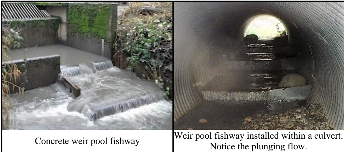
Figure 8.3. Photographic examples of weir pool fishway designs.
