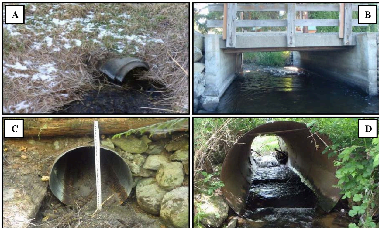
Figure 3.5. Examples of culvert construction materials. A) Precast concrete (PCC), B) Cast-in-place concrete (CPC), C) Corrugated Steel (CST), D) Smooth Steel (SST)
