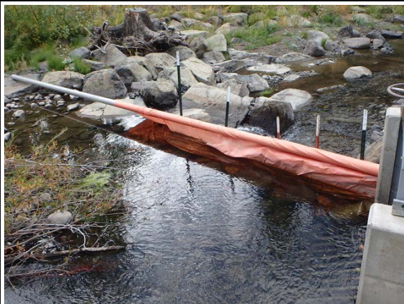
A full span seasonal dam (check structure) for irrigation.
