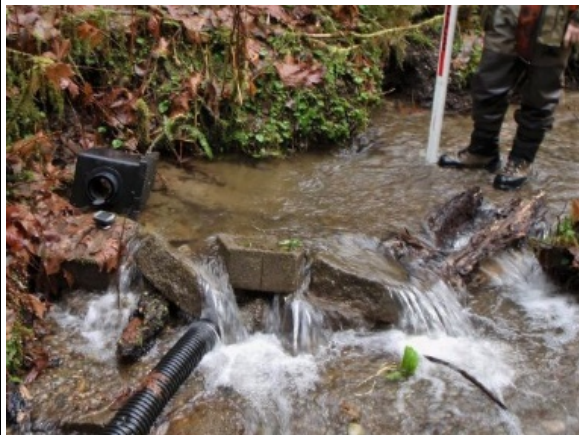
A partially spanning dam with an abandoned water surface diversion and no outlet type.
