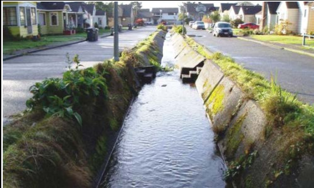
Flume – An artificial stream channel built to transport water, or transport materials using flowing water. Flumes include aqueducts and canals.
