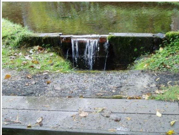
A full span concrete dam with a flashboard riser outlet type.
