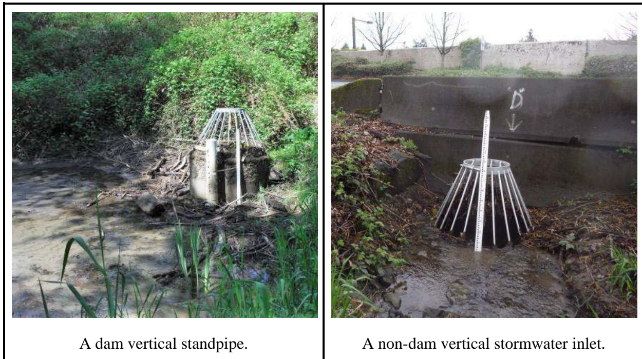
Figure 5.1. Photographic examples of dam standpipe, and non-dam vertical stormwater inlet. The dam standpipe on the left was designed for water detention, allowing debris and sediment to settle, and to constrain stormwater runoff. The non-dam stormwater inlet on the right was not installed to impound water. It was likely installed to access previously existing, underground stormwater management infrastructure; its primary purpose is water conveyance.
