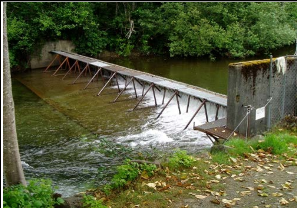
Hatchery Rack – A weir that functions to block, divert, or trap fish, for hatchery or other use.
