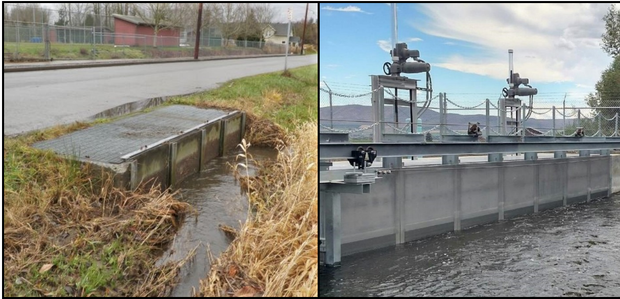
Figure 9.7. Photographs of vertical plate screens.
