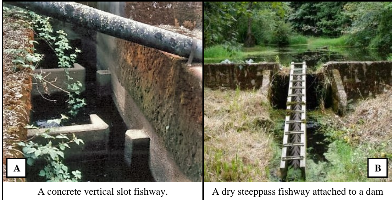
Figure 8.5. Photographic examples of vertical slot (A), and steeppass (B) fishway designs.
