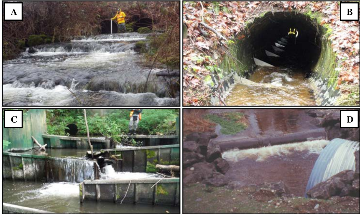
Figure 3.17. Examples of culverts with fishways. Fishways may be located upstream, downstream, or within a culvert and are intended to facilitate fish passage up to, through, and away from the structure. A) A rock streambed control fishway at downstream end of dual culverts. B) Culvert with interior metal baffles. C) Weir pool fishway at downstream end of culvert. D) Log streambed control fishway at upstream end of culvert.
