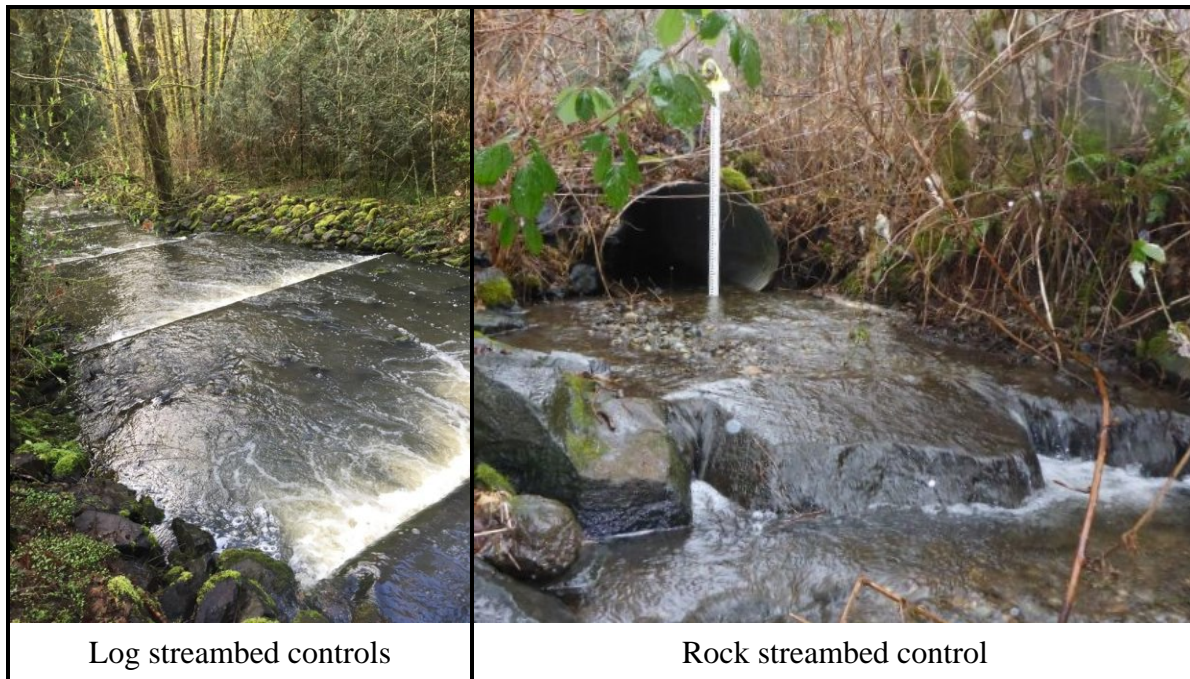
Figure 8.7. Photographic examples of streambed control materials.
