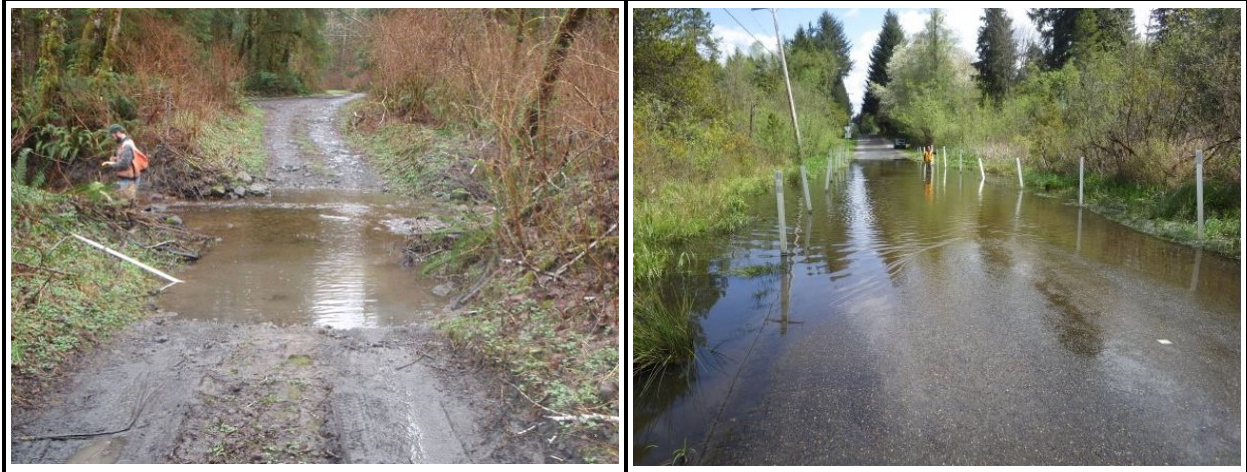
Figure 4.3. Photographic examples of ford non-culvert crossings.
