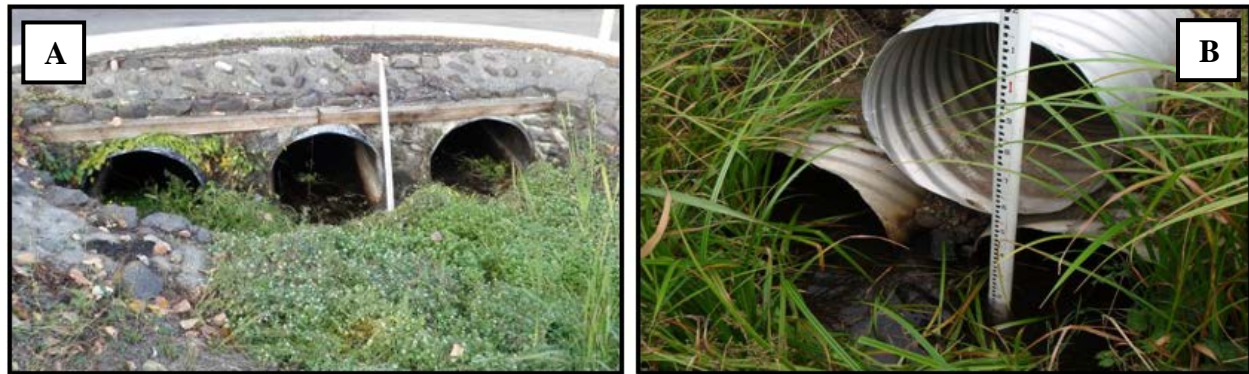
Figure 3.4. Photo examples of multiple culverts at a single water crossing. A) three non-overflow culverts. The culvert number for the culvert nearest the left bank is 1.3, the middle culvert number is 2.3, and the culvert number for the culvert nearest the right bank is 3.3. B) two non-overflow culverts and one overflow culvert. The culvert number for the culvert nearest the left bank is 1.2 and the culvert number for the culvert nearest the right bank is 2.2. The top middle culvert's size, shape, and material are described in the comments, e.g., '0.61 m round corrugated steel overflow culvert', and is not assessed for fish passage.
