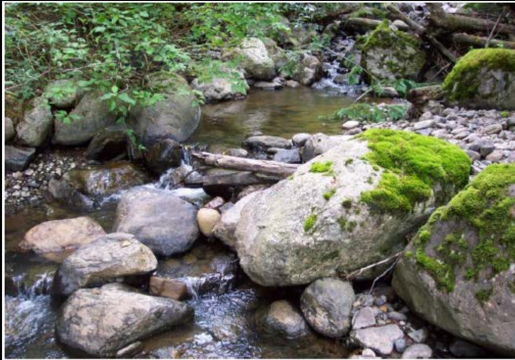
Roughened Channels – A channel constructed from boulder sized roughness elements placed in a pattern to increase roughness. Roughened channels control gradient, reduce velocity, or serve other restoration purposes.
