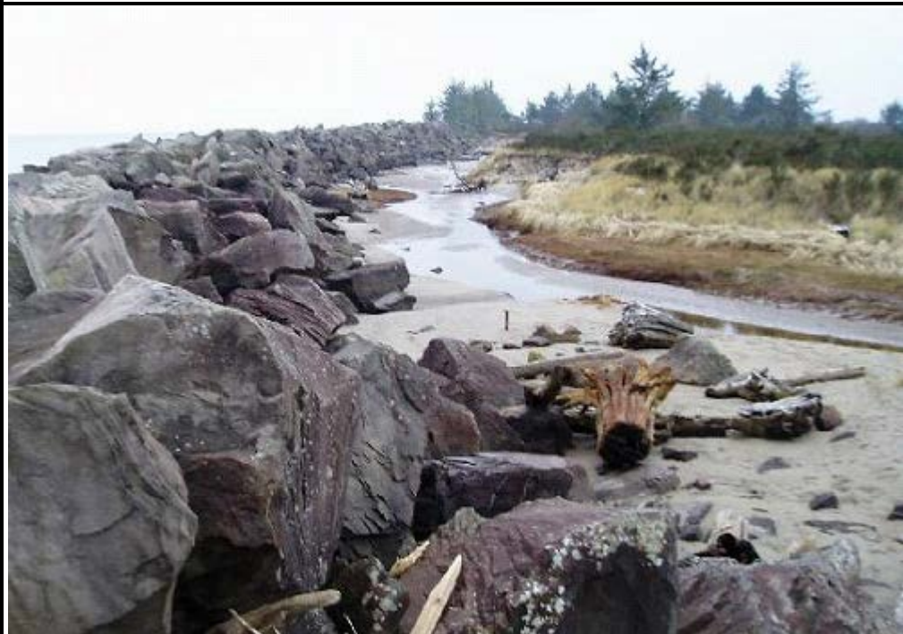
Dike/Levee – An embankment built to prevent flooding from other waterbodies. Jetties that act as barriers are also classified as a Dike/Levee.
