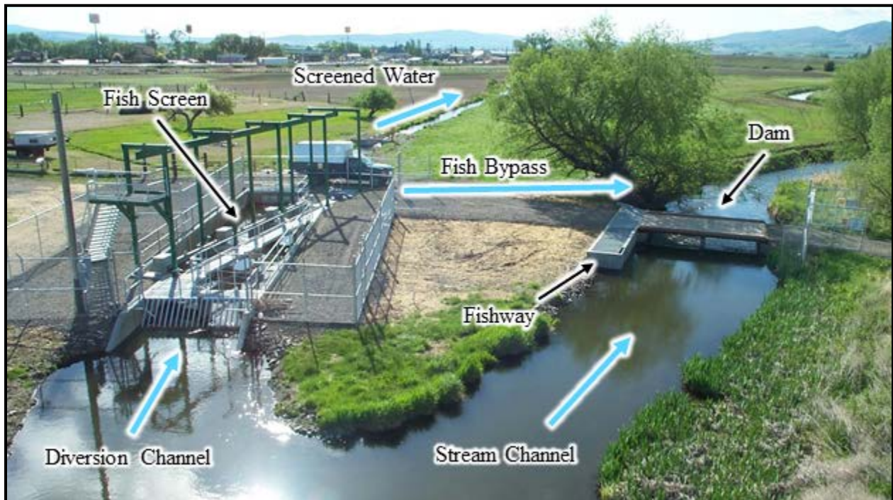
Figure 9.1. Photographs of a surface water diversion and associated fish passage feature. The image depicts the screened diversion channel, the associated fish passage feature (dam), attached fishway, and bypass channel.
