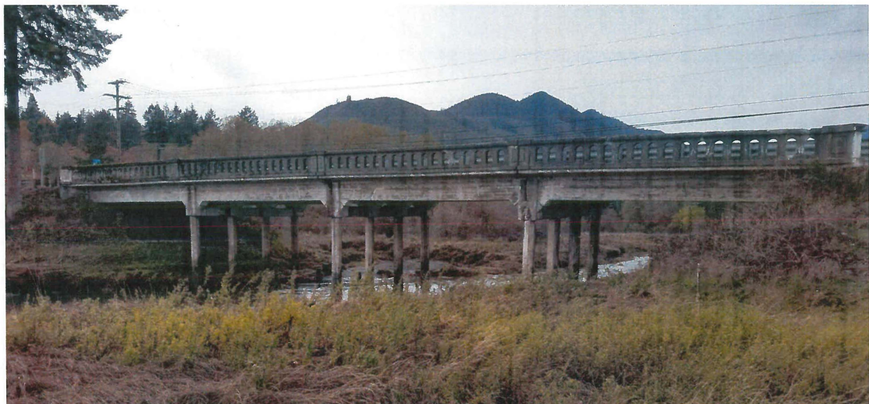
Figure 2: Elevation view of Duckabush River Slough Bridge No. 101/265, looking upstream
