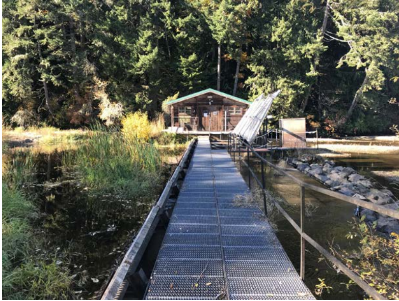
WDFW Fish weir – Big Beef Creek Unit. Photo by Darric Lowery.
