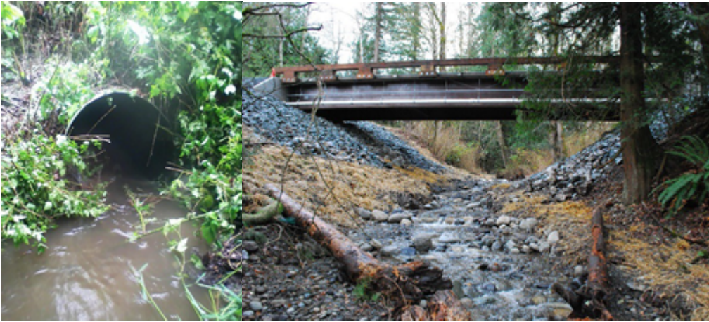
After - New bridge installation
