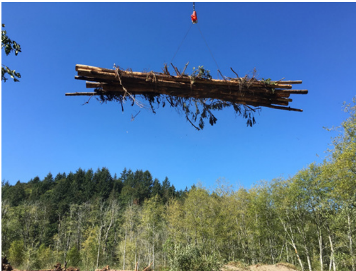
Restoration work on the Manastash.
